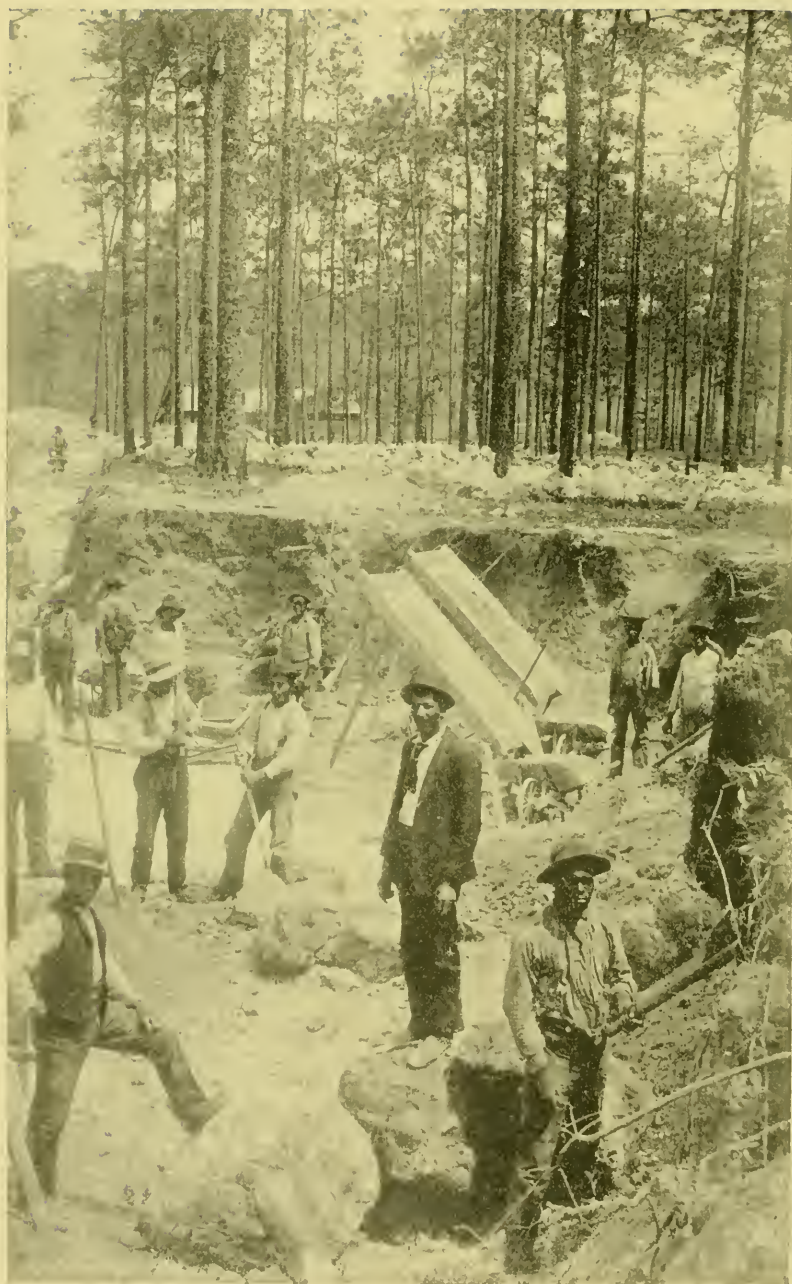
FLORIDA ROCK-PHOSPHATE MINING. Working in "boulder" material after removal of top soil.
