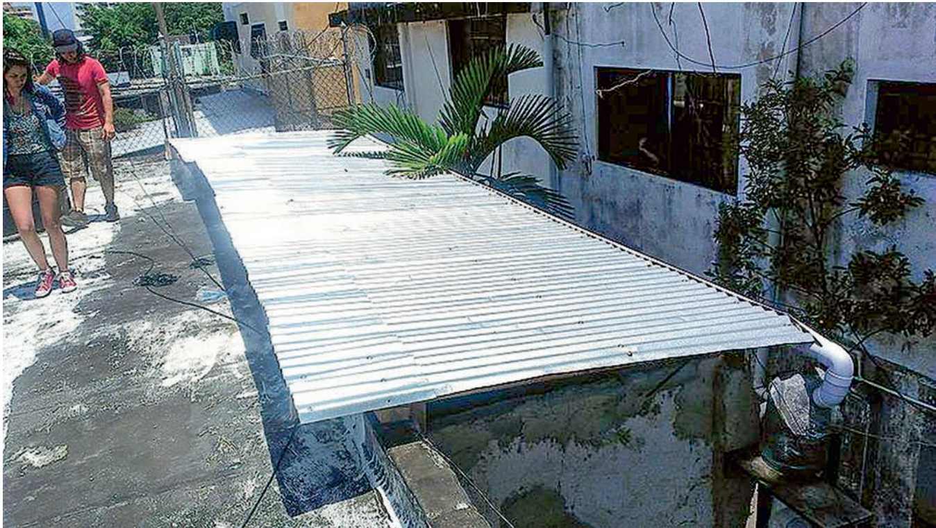
Figure 2-5 Corrugated metal roof in Santo Domingo, Dominican Republic. proppedia.org/La_Yuca_rainwater_2014
