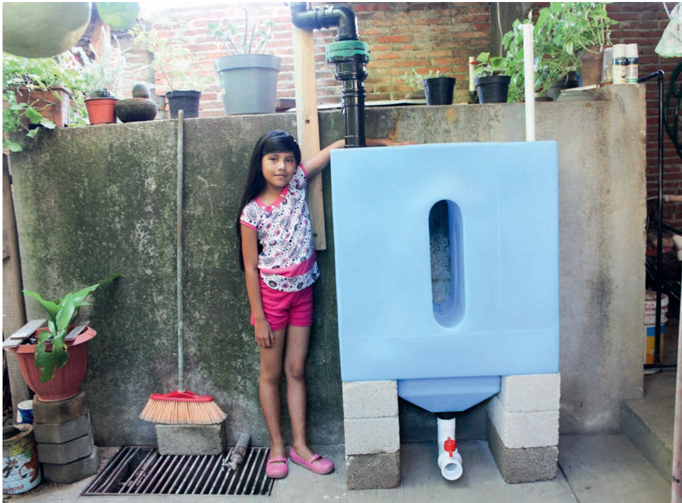
Figure 5-14 Rainwater harvesting system at a home in southern Mexico City with a Tlaloque first-flush by Isla Urbana. Provides six months of total water autonomy per year. appropedia.org/Isla_Urbana
