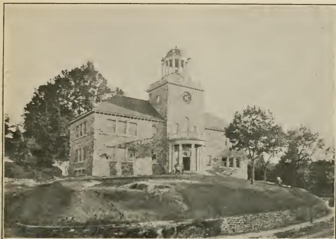
Canal Street School Building, Brattleboro, Vt.
