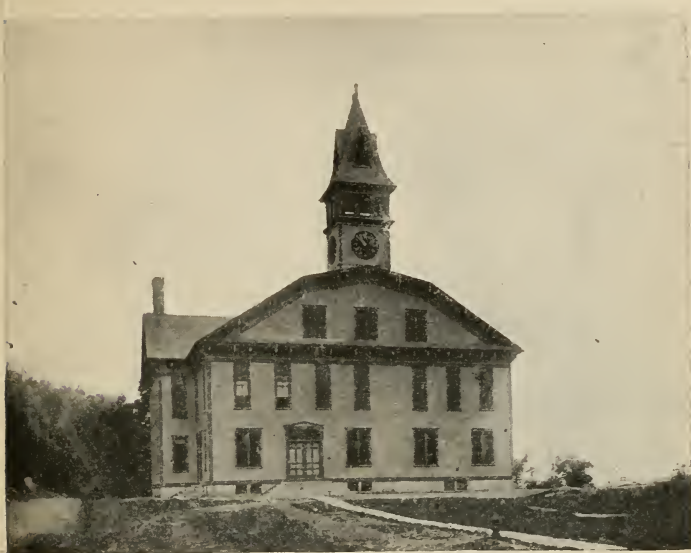
Proctor High School Building Rutland County
