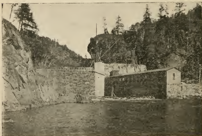
Bolton Falls Dam and Electric Light Plant on Winooski River
