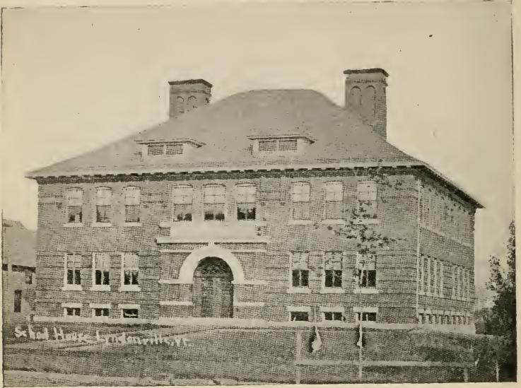
Lyndonville School Building Caledonia County
