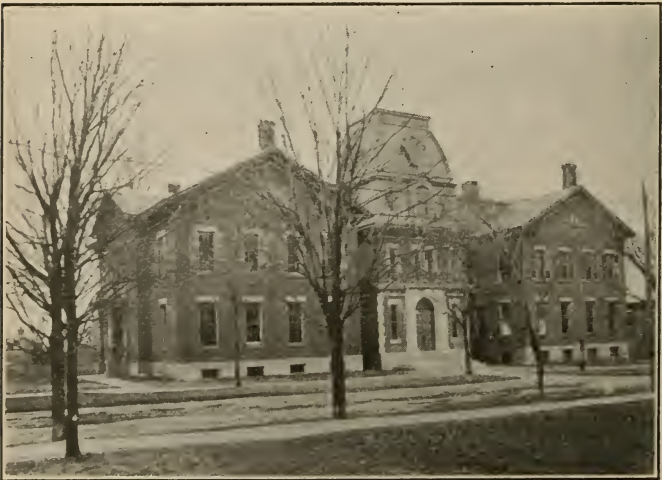
Rutland High School Building Rutland County
