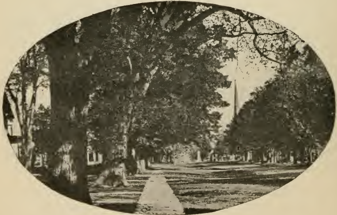
Main Street of Manchester, Bennington County.
