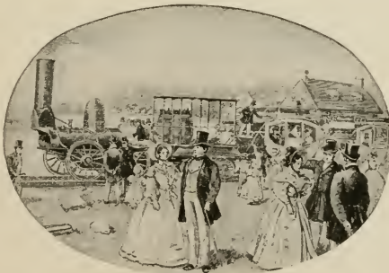
Early transportation—first railway train
