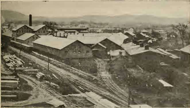
The Howe Scale Company Works, Rutland.
