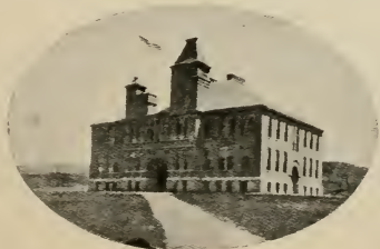
Waterbury High and Graded School Building.
