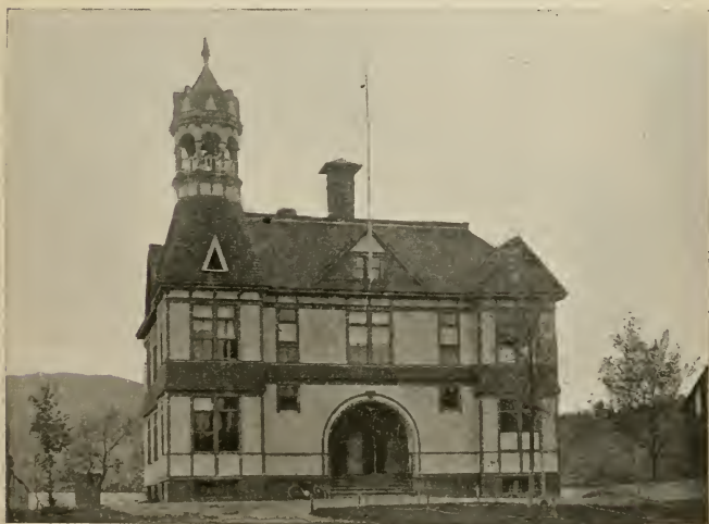
South Royalton High School Building Windsor County
