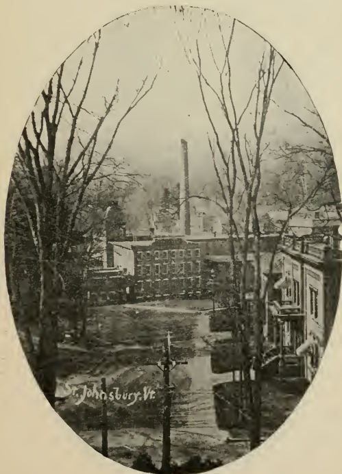
The Fairbanks Company Scale Works, St. Johnsbury.
