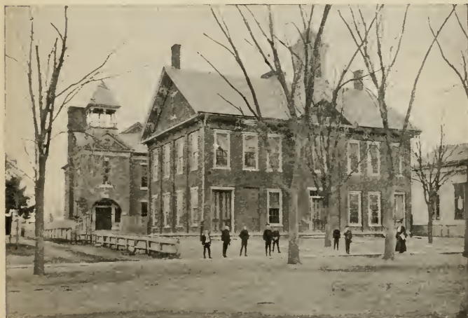
Fair Haven High and Graded School Building Rutland County
