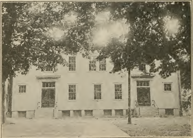
Wallingford High and Graded School Building Rutland County
