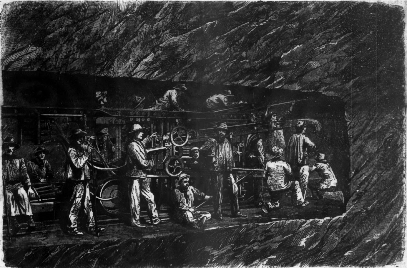
BORING THE MONT CENIS TUNNEL.
