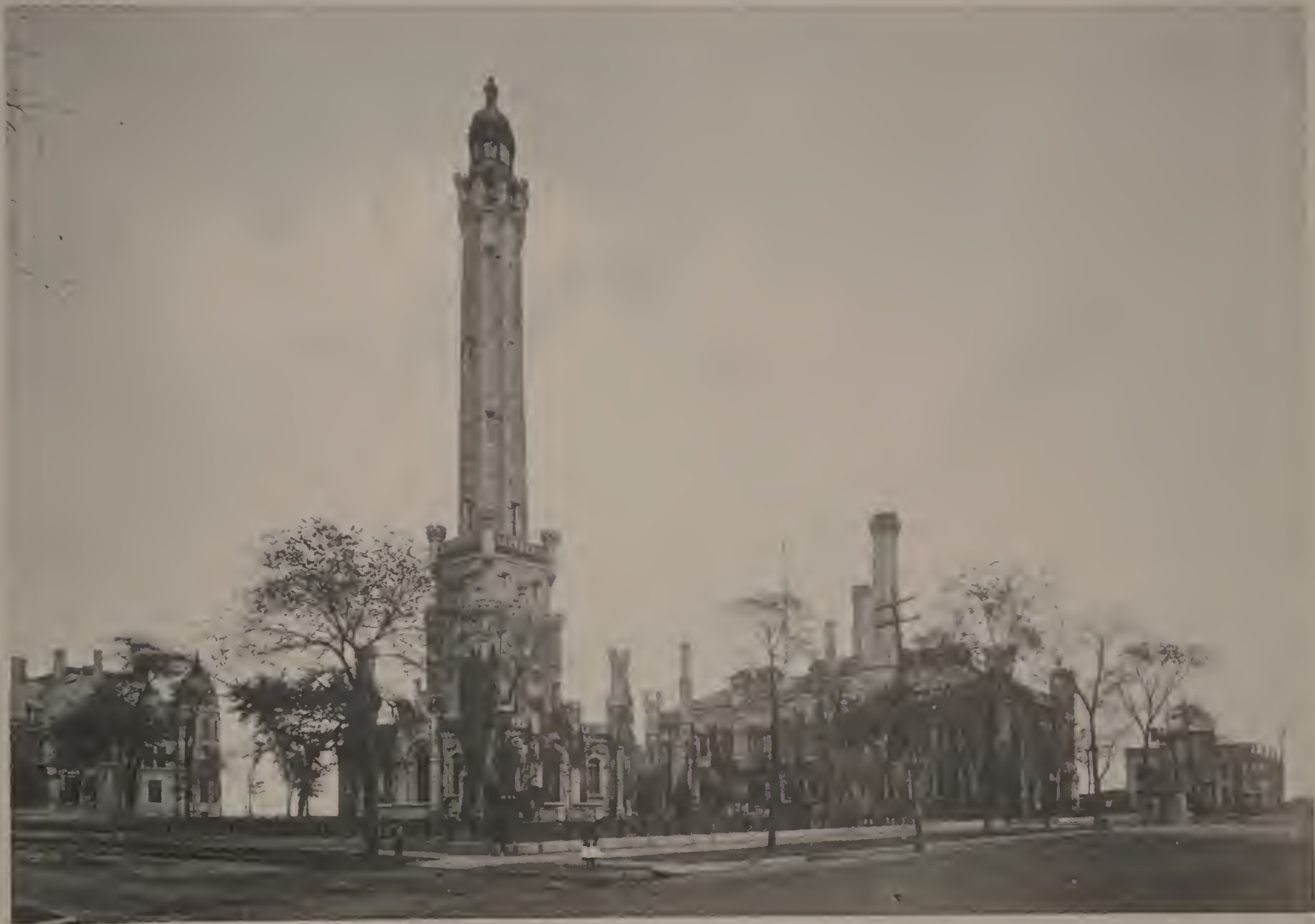
NORTH SIDE WATER WORKS.
