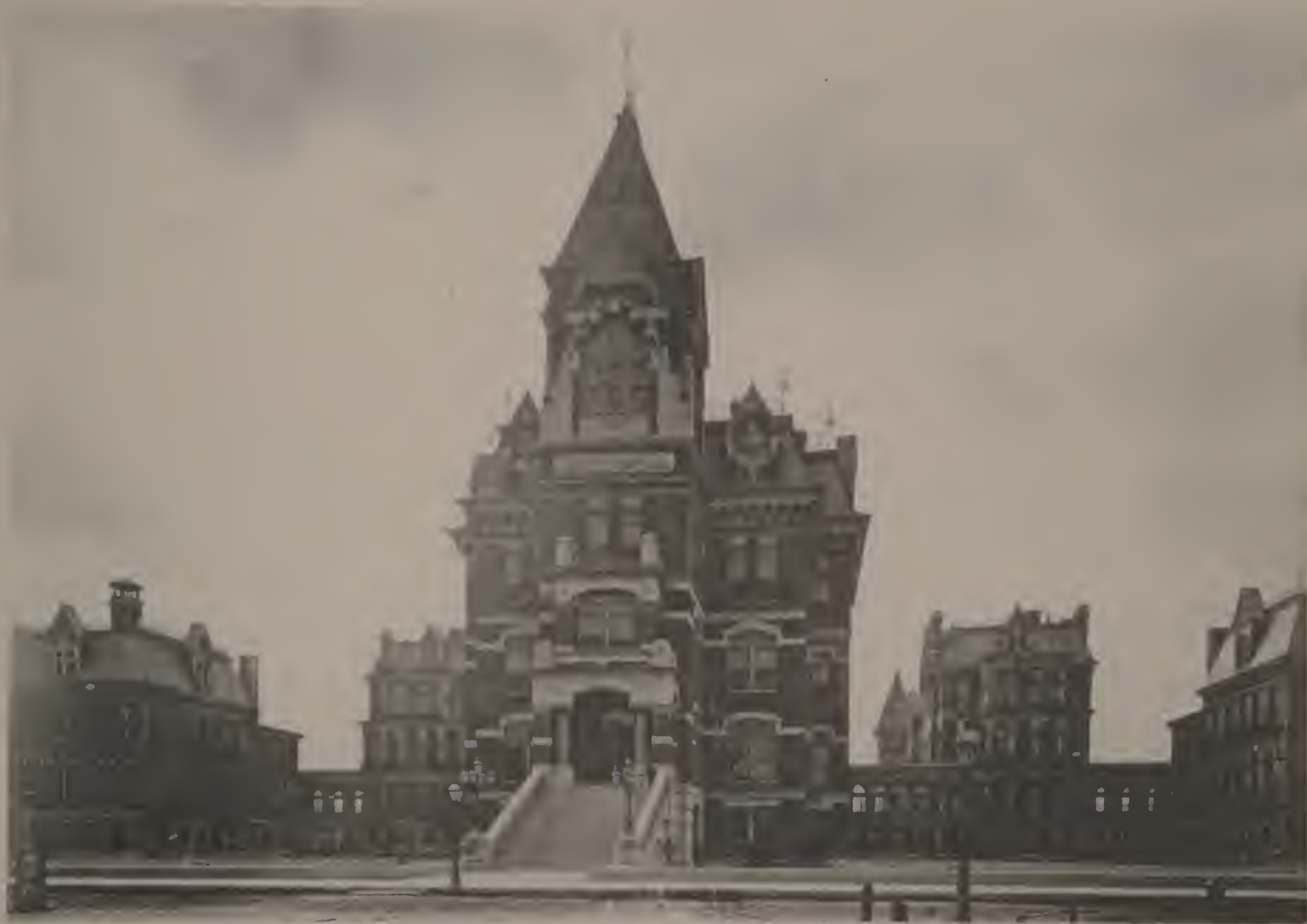
COOK COUNTY HOSPITAL.
