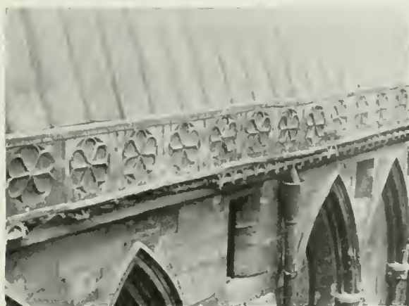
FIG. 189.—Parapet Gutter, Lincoln Cathedral.
