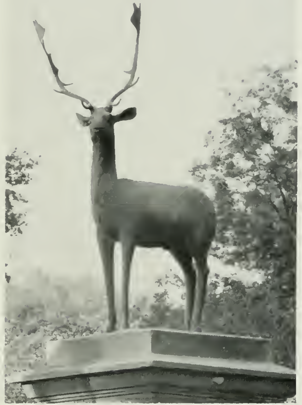
FIG. 287.—Stag on Gate Pier, Albert Gate.
