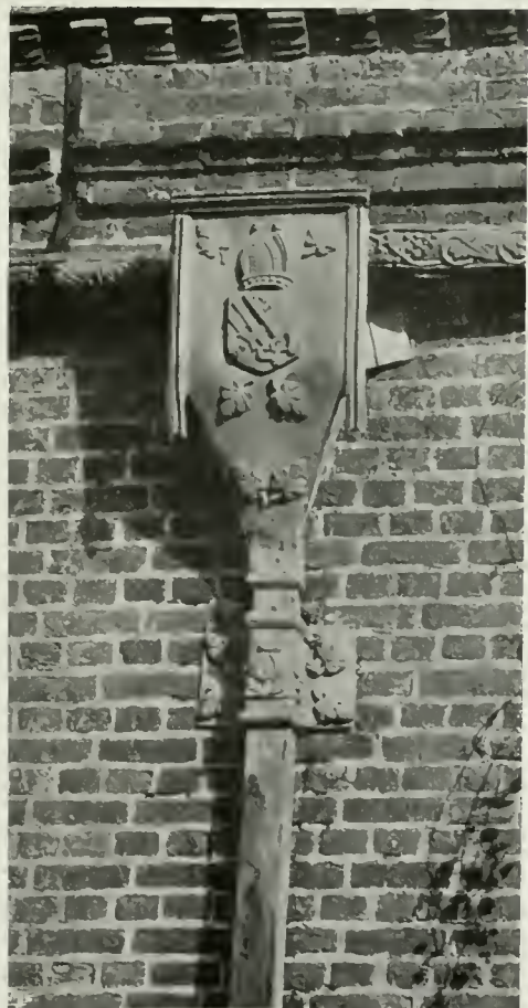
FIGS. 58-60.—PIPE-HEADS, GUTTER, AND APRON, DOME ALLEY, WINCHESTER.
