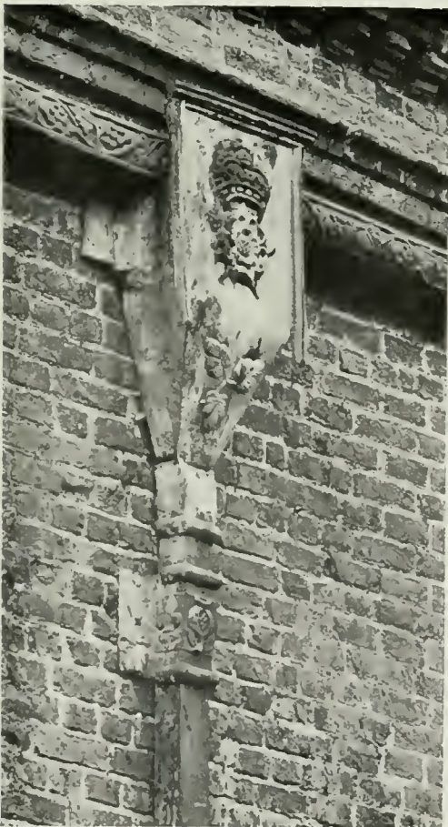
FIGS. 58-60.—PIPE-HEADS, GUTTER, AND APRON, DOME ALLEY, WINCHESTER.
