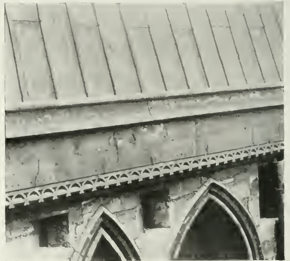
FIG. 191.—Leaded Parapet, Lincoln Cathedral.
