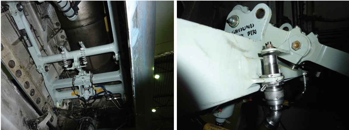
Figure 15: stabilizer brace assembly (left) with gear proximity sensors and target plate (right).
