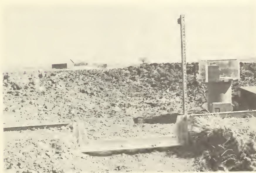
Figure 8.—Cipolletti weir installation for measuring surface runoff.
