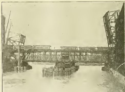
World's biggest jack-knife bridge constructed at Chicago, Ill. Copyright, 1915, Hearst-Selig News Pictorial.
