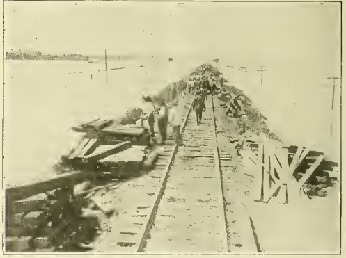
Working to save flood swept railroad in Kansas. Copyright, 1915, by Hearst-Selig News Pictorial.
