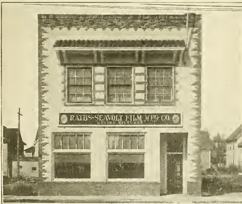
Rath and Seavolt's new laboratory and factory in St. Paul, Minn., which was fully described in last week's issue of MOTOGRAPHY.
