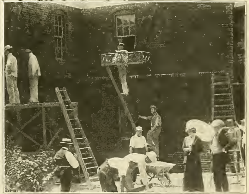
Another scene of the brick wall.
