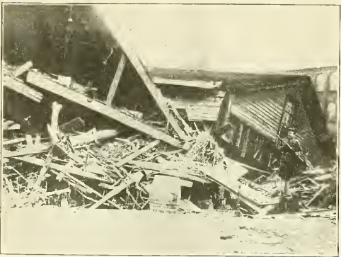
Wreckage caused by floods at Erie, Pa. Copyright, 1915, Hearst Selig News Pictorial.
