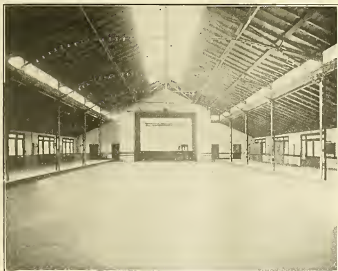
Interior of studio building, now being remodeled.
