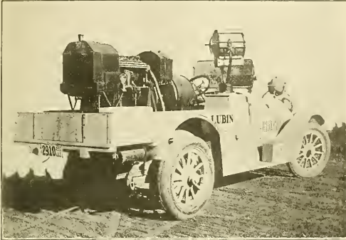
Lubin's portable lighting plant.
