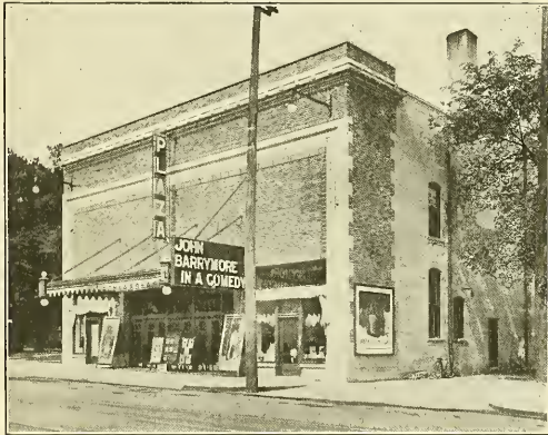
Exterior of the Plaza Theater, Waterloo, Ia.
