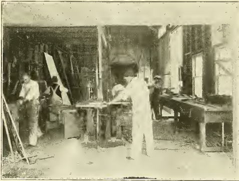
The carpenter shop is one of the busiest places in the entire plant.
