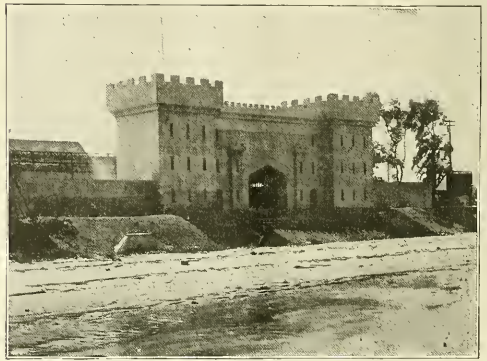
This massive gate impresses all who seek entrance to the studio and is useful besides.
