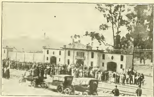
Crowd in front of building that was constructed and burned to make a single scene in a coming Keystone-Triangle feature.
