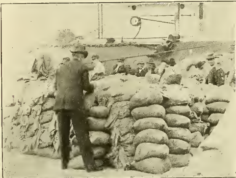
Sand bags used in stability test on S. S. Christopher Columbus, at Chicago, Ill. Copyright, 1915, Pathe News.
