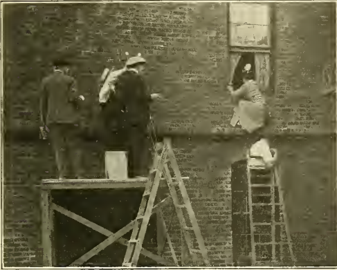
Brick wall erected for scene that will last for five seconds.
