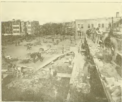
Constructing Essanay's new studio, 350x175 feet, said to be the largest indoor artificially lighted studio in the world.
