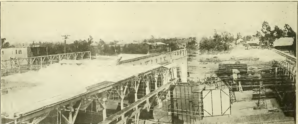
A comprehensive bird's-eye view of the Balboa plant showing the arrangement
