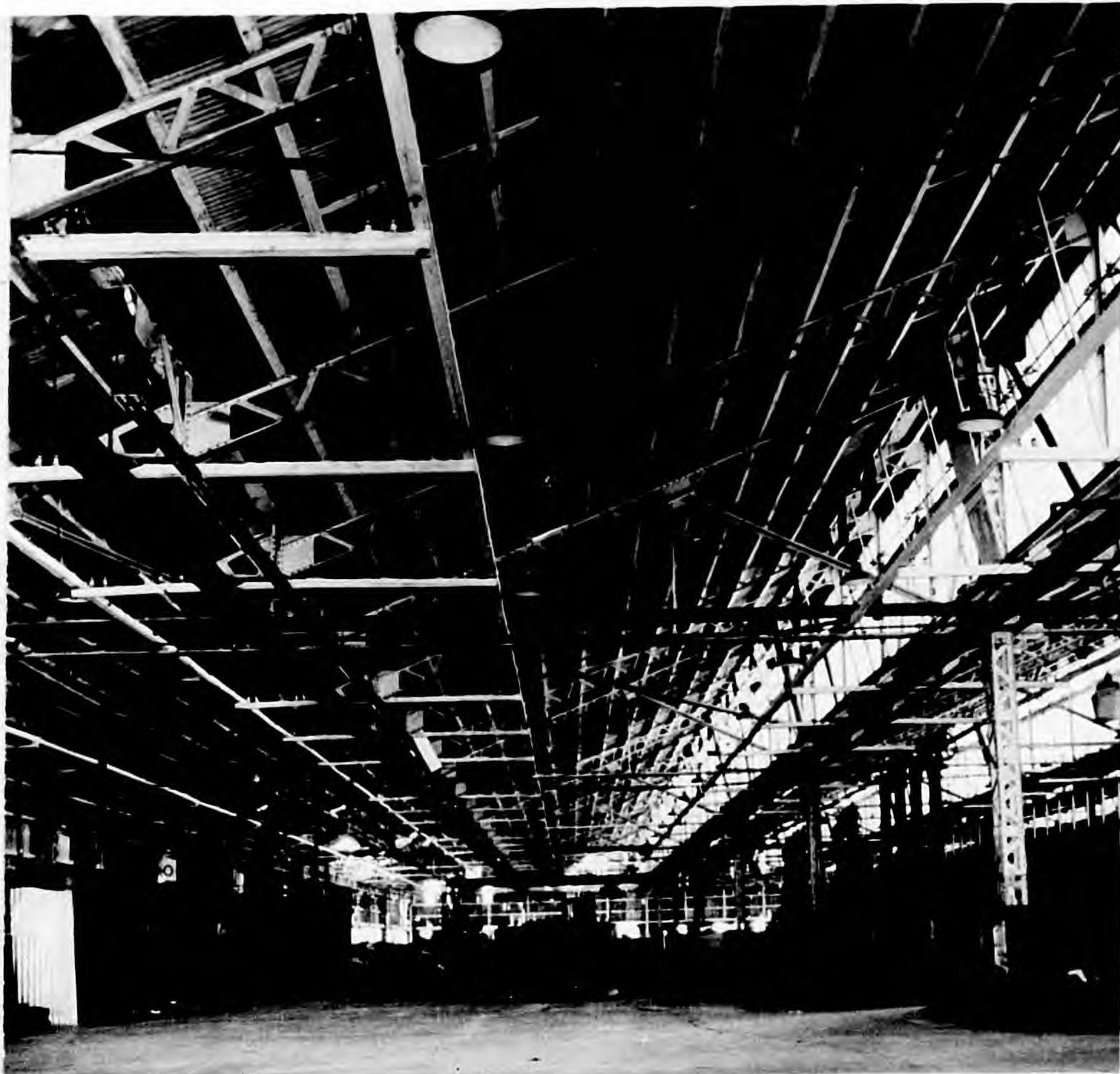
Photo 1 - Typical roof construction in Bldg 1, showing details in roof which has not been disturbed by bomb- ing.
