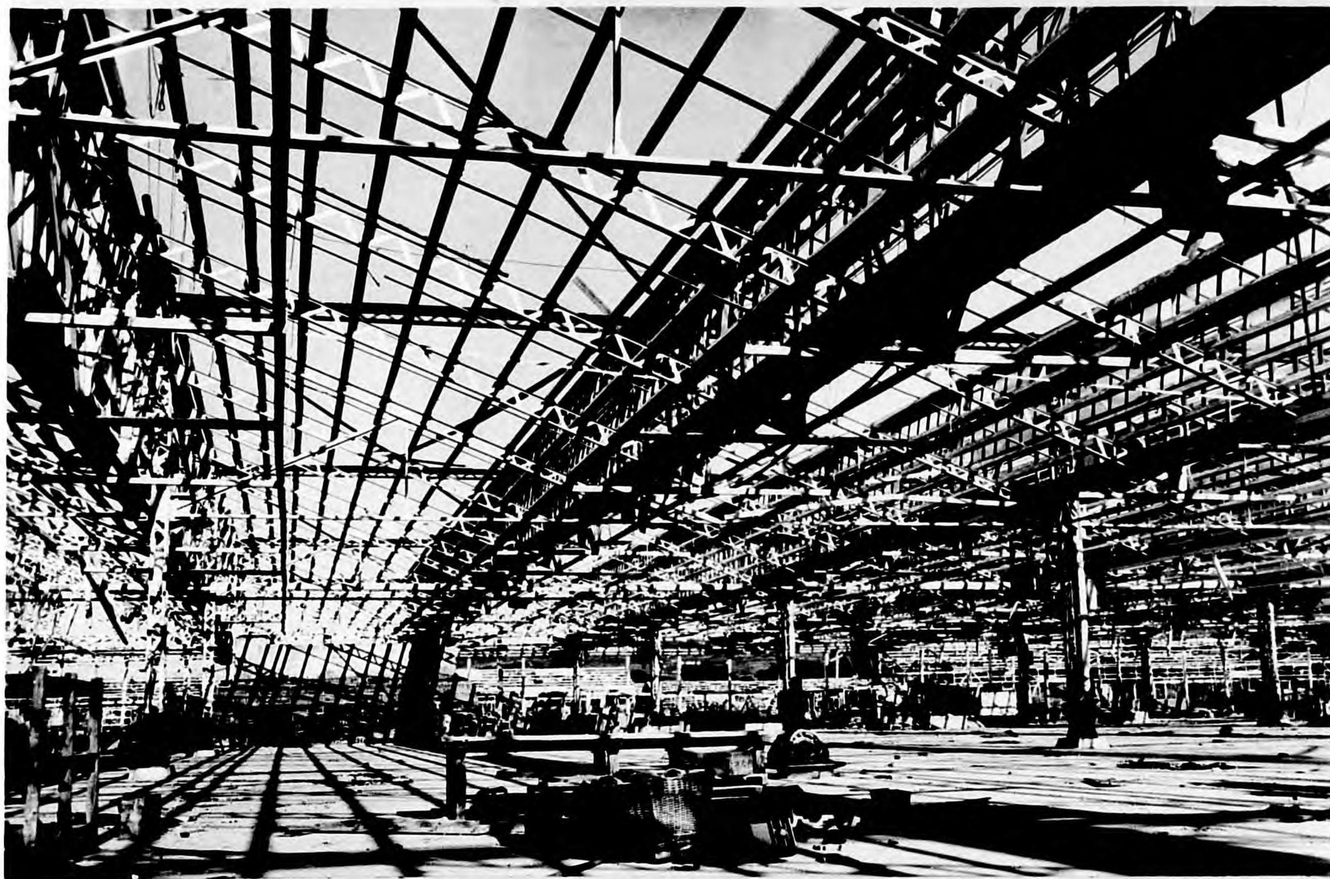
Photo 2 - Roof construction in Bldg 1, showing bare trusses where roof covering and glass have been completely removed.
