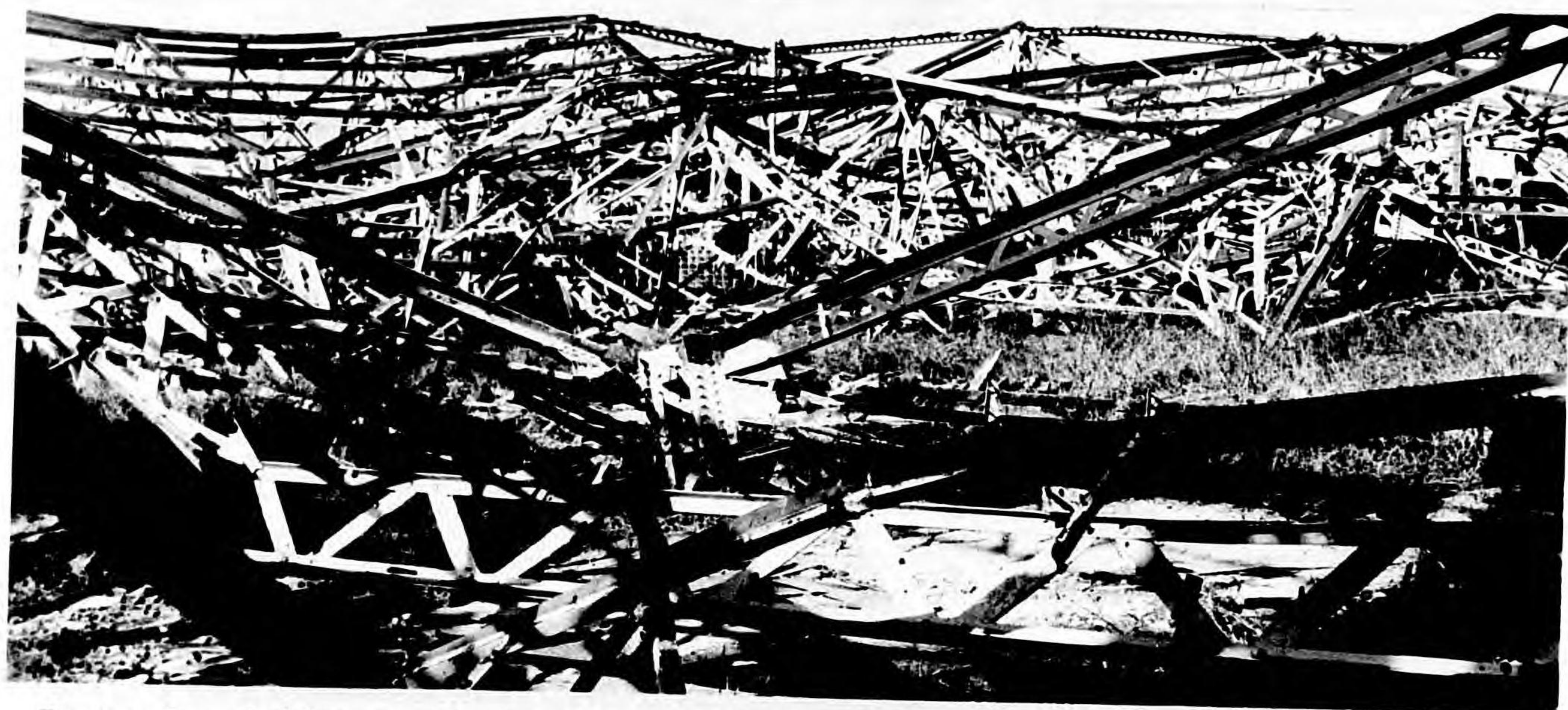
Photo 5 - Collapse of the shop roof occasioned by the direct hit of Bomb 12. This damage was increased by effects of Bombs 10 and 11, which detonated to the right of the picture.
