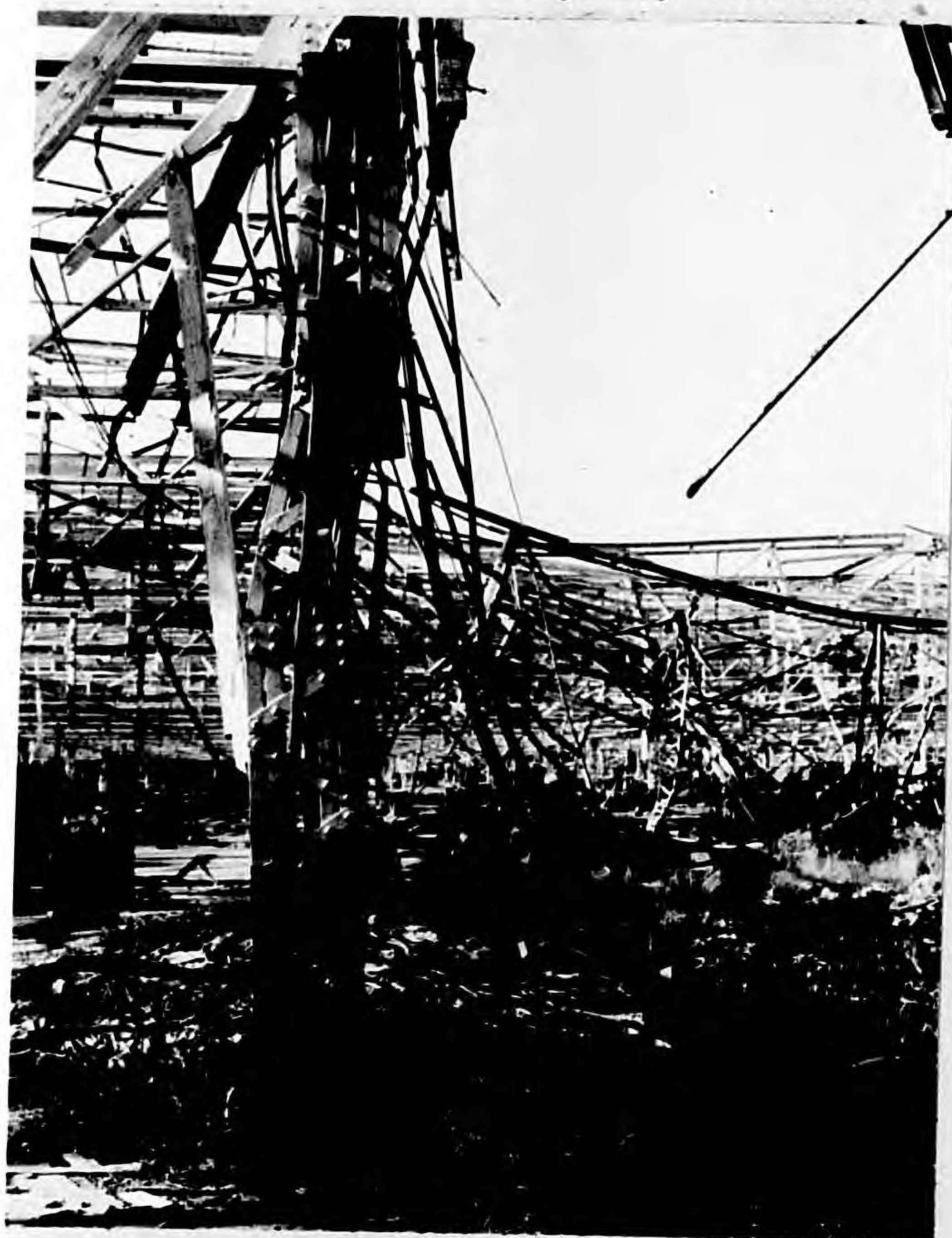
Photo 13 - In the foreground is Column 11-D, showing the effect of earth shock, blast and strain on a typical supporting column.
