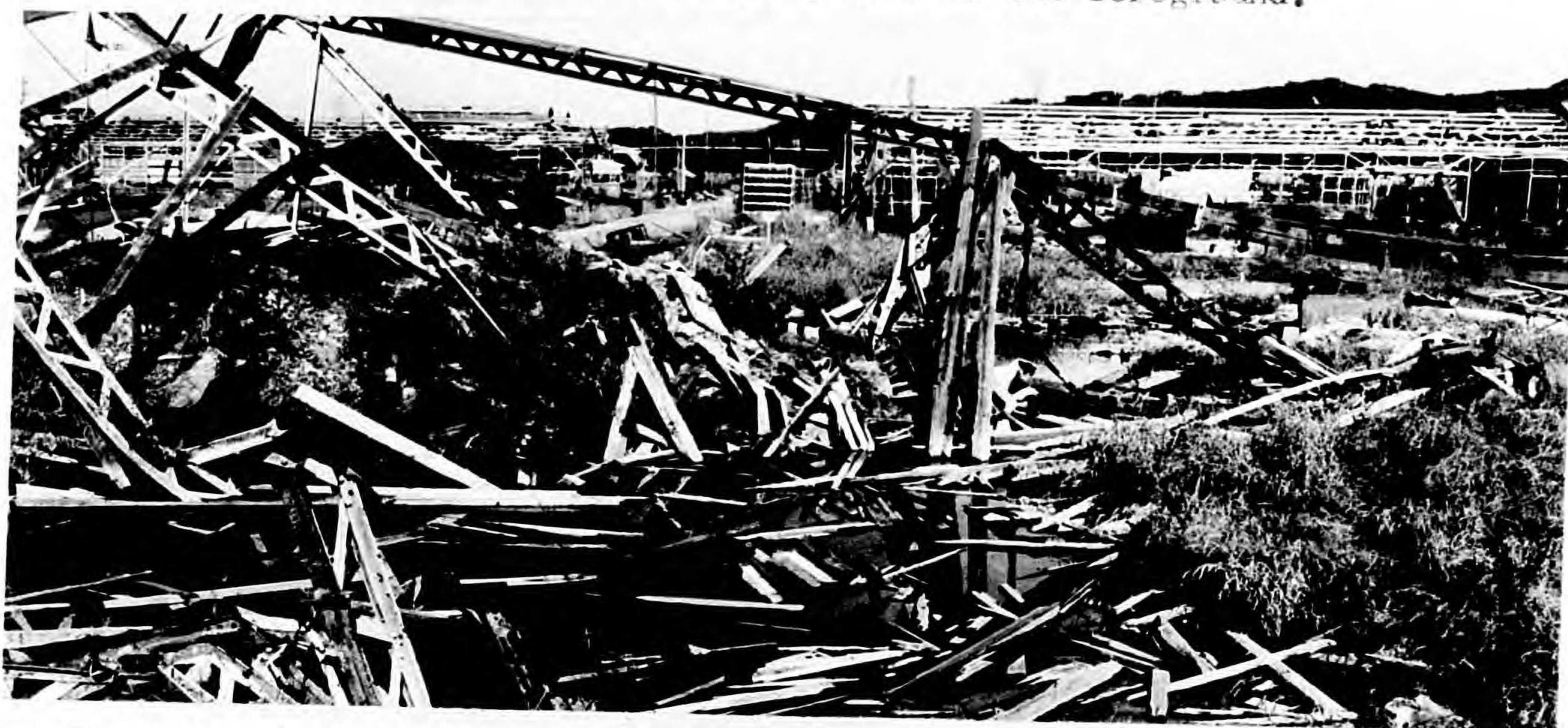
Photo 4 - Damage from Bomb 11 (foreground), a direct hit, and Bomb 10 (background), a near miss. This portion of Bldg 1 was destroyed.
