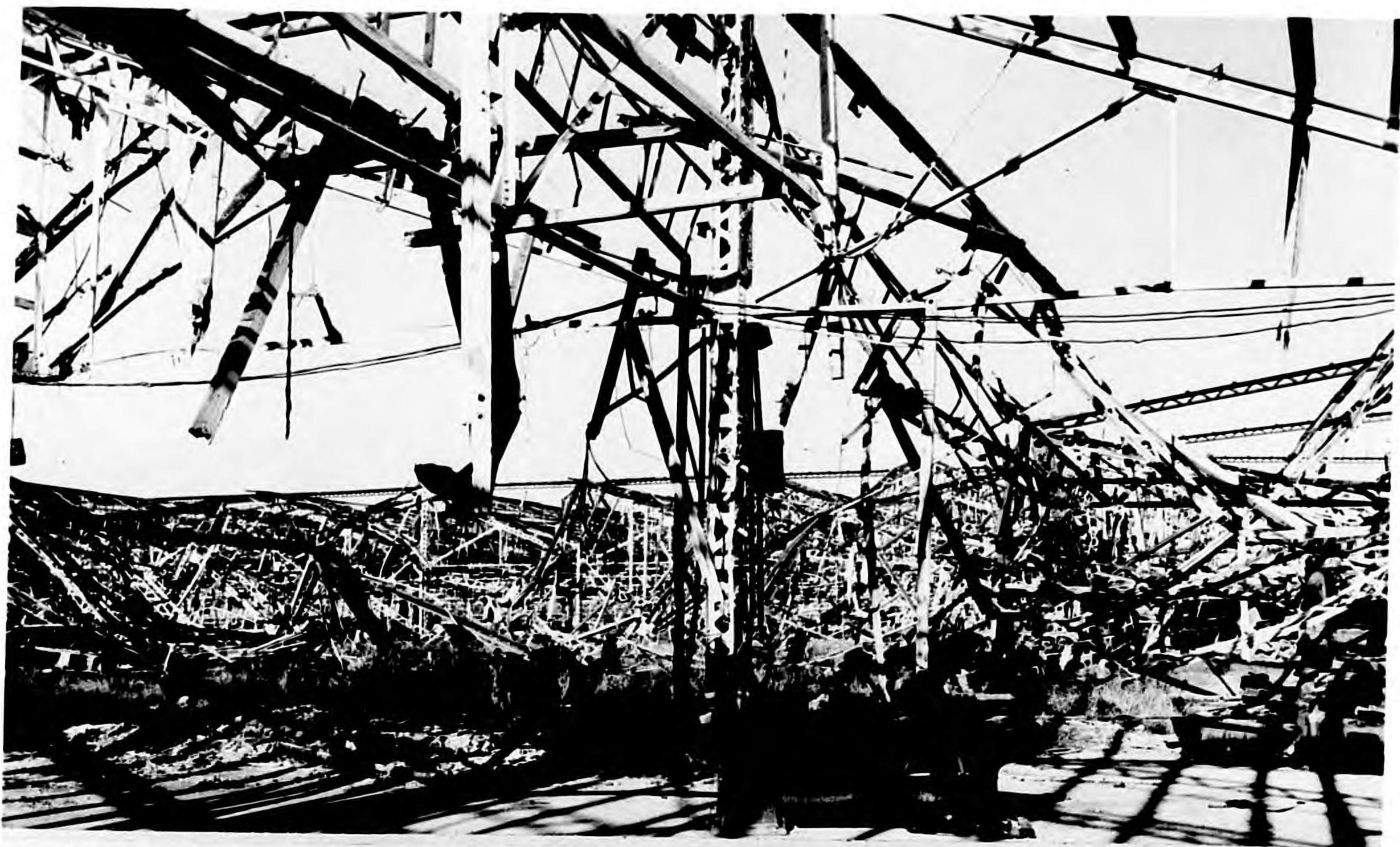
Photo 12 - A general view of the complete collapse of the shop structure caused by Bombs 16, 17, and 18.
