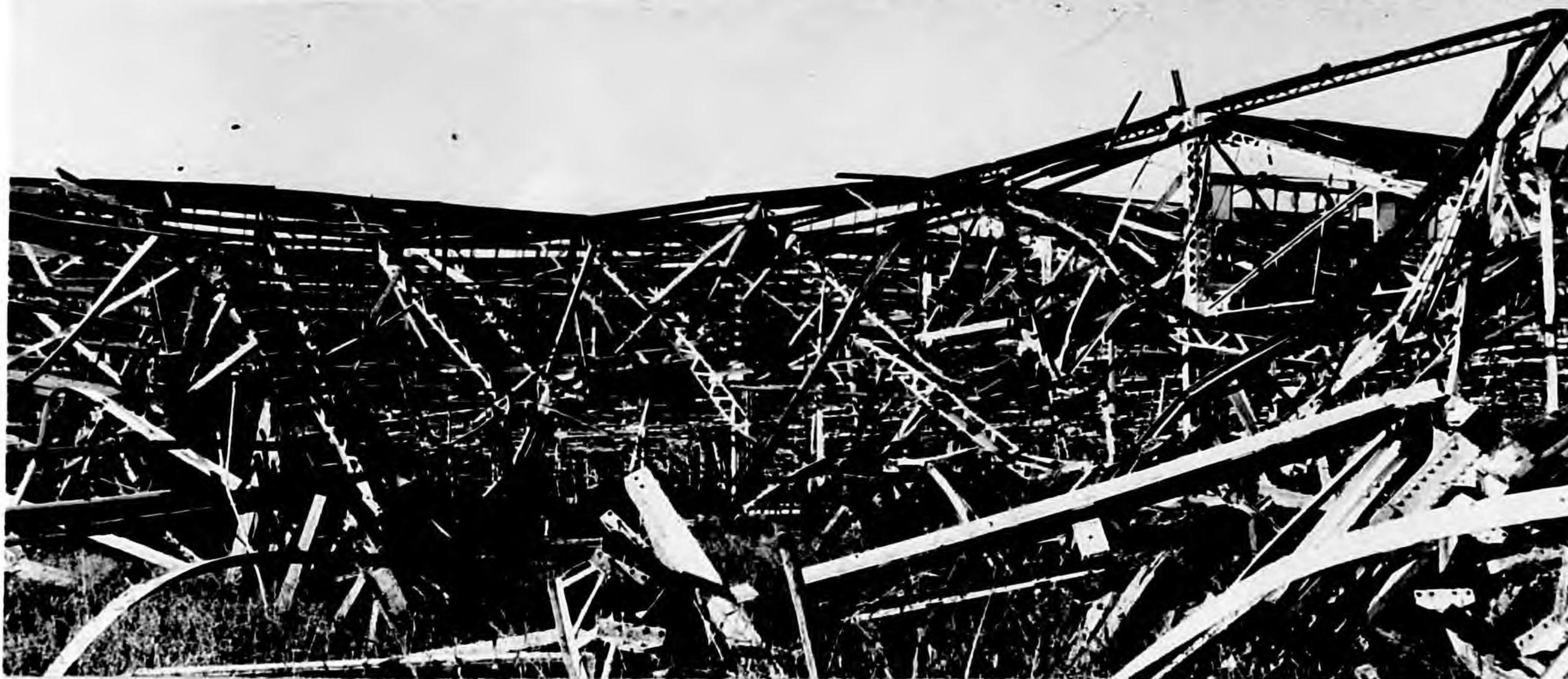
Photo 19 - A partial view of damage caused by Bombs 16 and 17. Weeds and grass tend to obscure craters and detail of damage at crater level.
