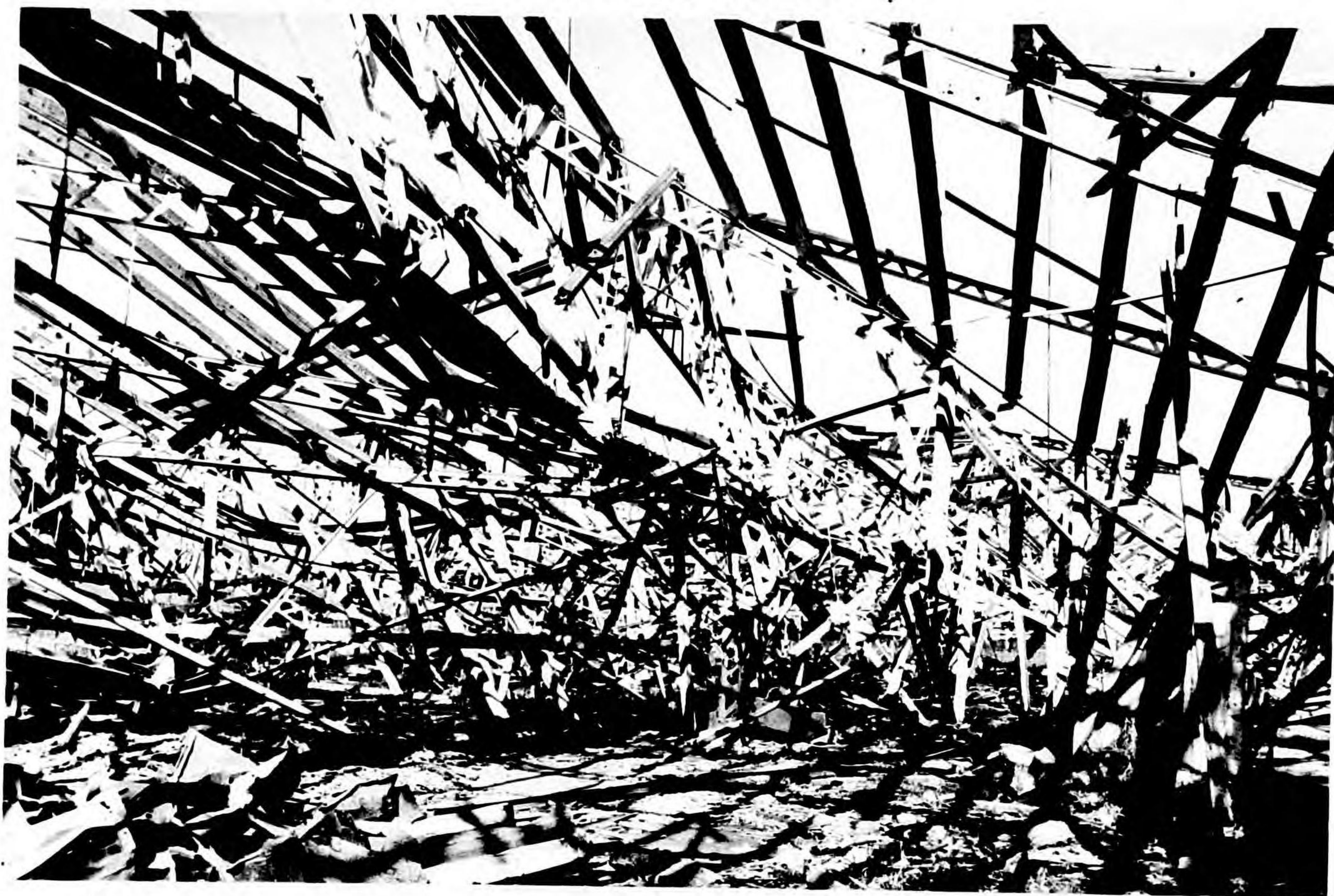
Photo 7 - In the foreground, tangled wreckage caused by Bomb 12. In the background, damage caused by Bombs 8 and 9.
