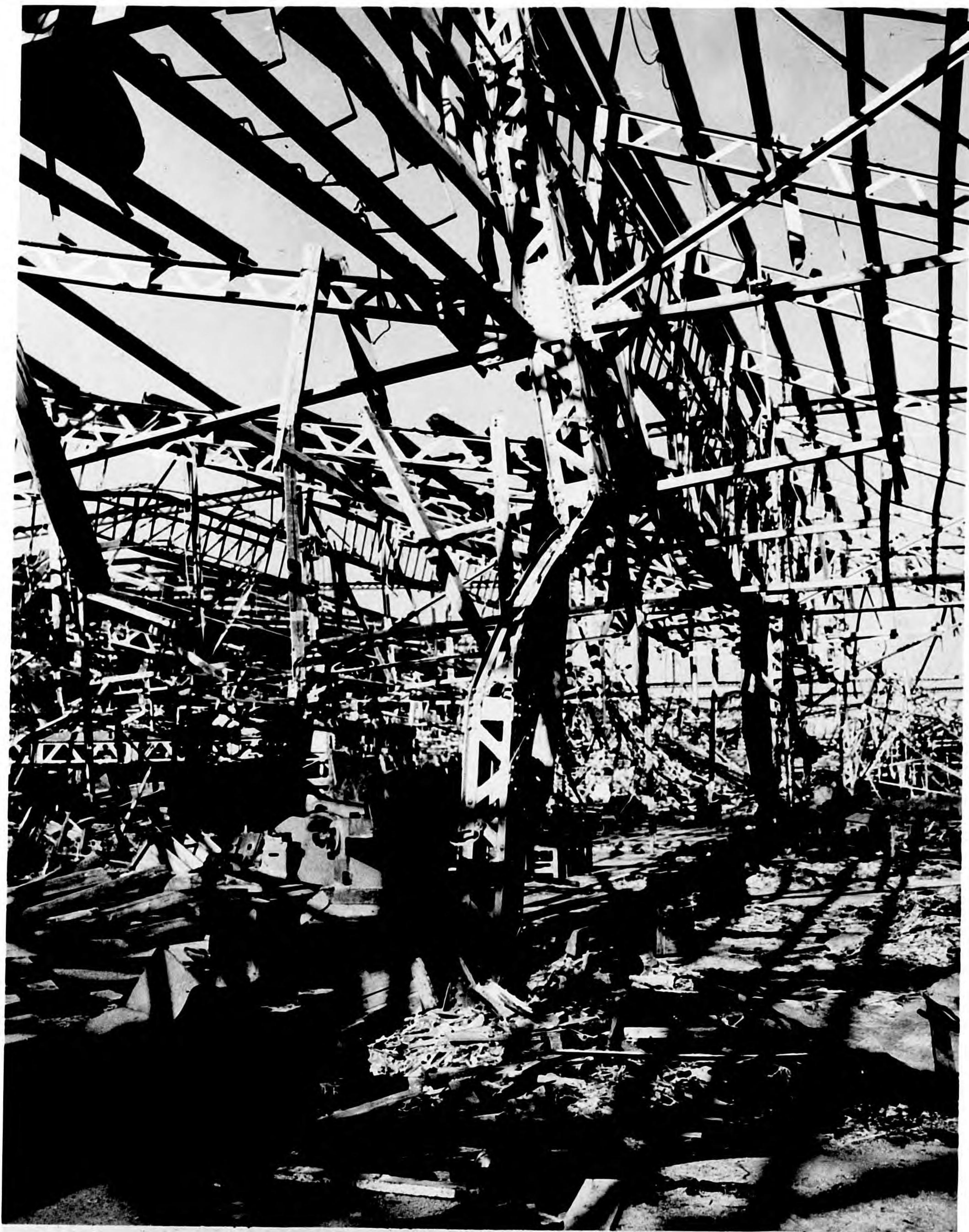
Photo 15 - Column 12-E shows the effect of earth shock and shifting of column footing as the column failed under compression.
