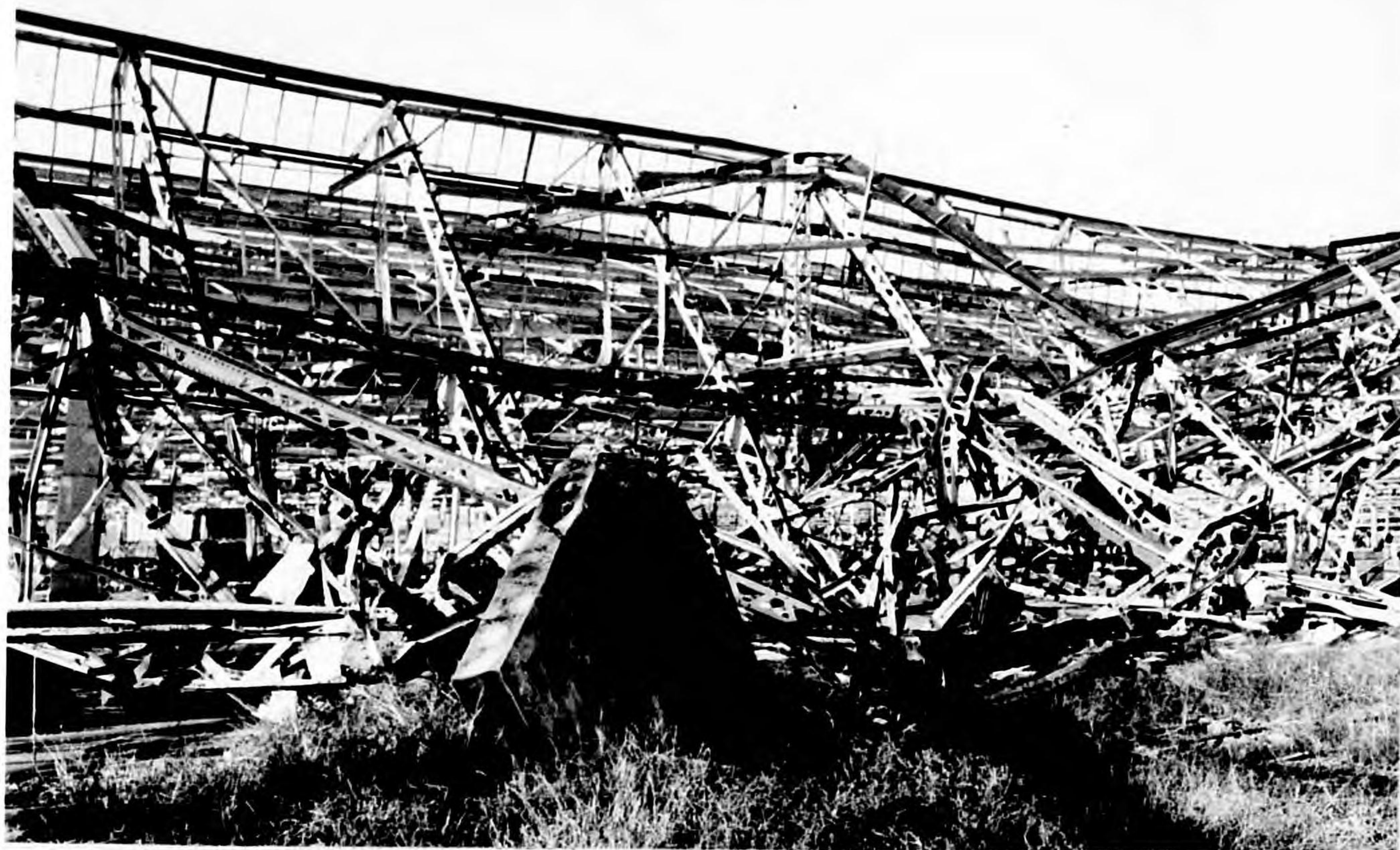
Photo 16 - In the center foreground is the footing of Column 11-E, upturned by Bomb 18, indicating the disruptive effect of this bomb. The background shows more of the overall damage effect of Bombs 16, 17, and 18.
