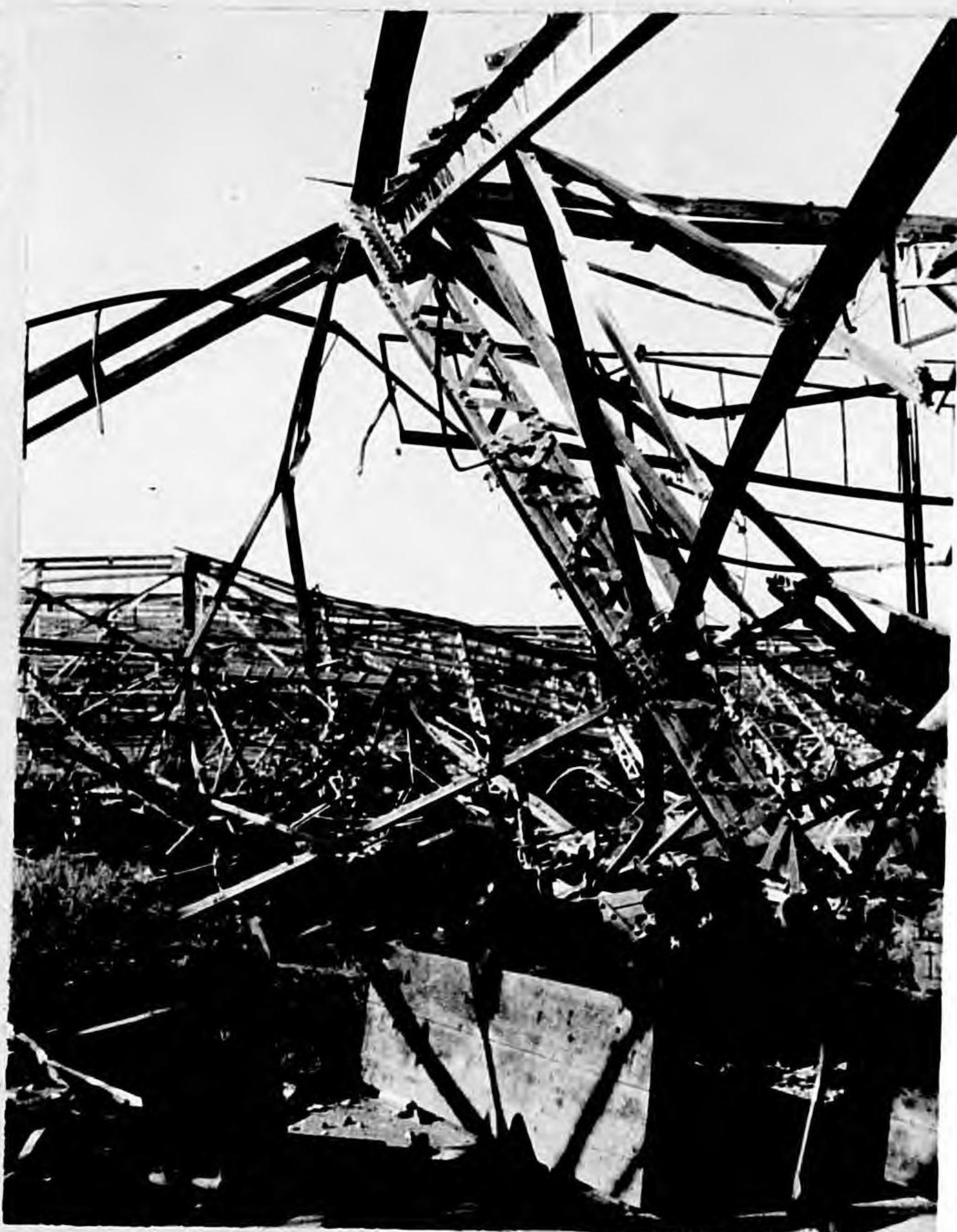
Photo 14 - In the foreground is Column 12-F sheared at the base by Bomb 18 and pushed over, causing partial collapse of the roof.
