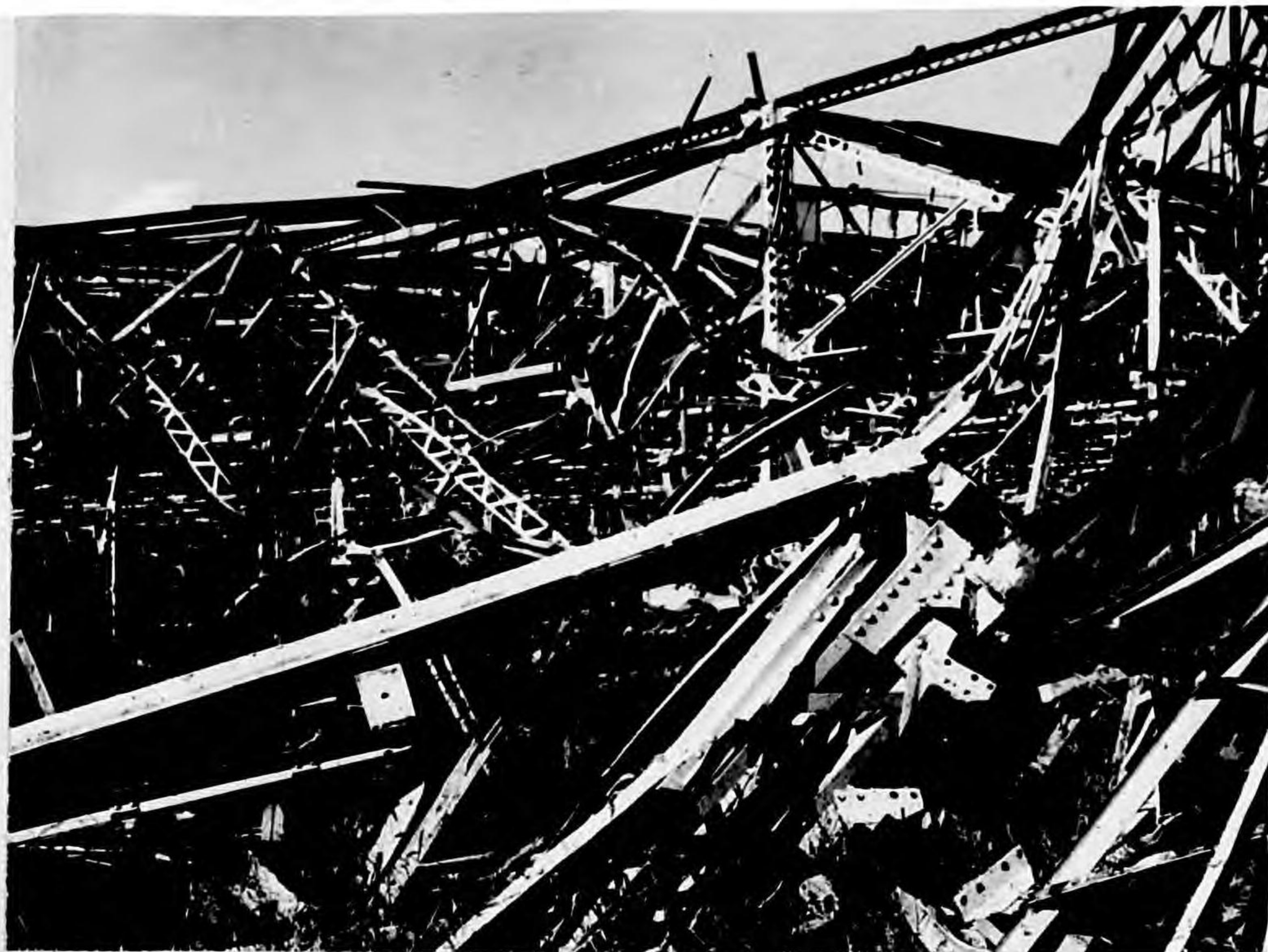
Photo 18 - Detail of failure of Column 10-F which was sheared approximately 4 inches from its base and shattered into scrap.
