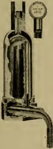
Figure 75. Type of air valves commonly used on radiators.
