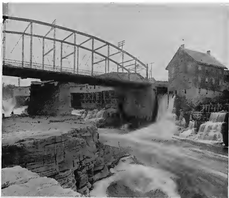
THE BRIDGE AT GLENS FALLS
