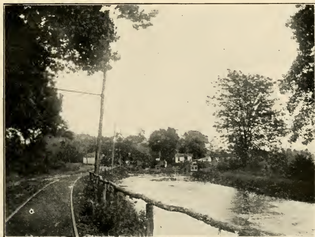
ROADWAY ALONG THE CANAL AT KINTNERSVILLE.
