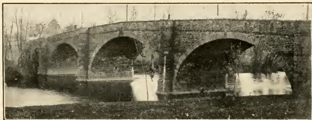
PERKIOMEN BRIDGE AT COLLEGEVILLE.
