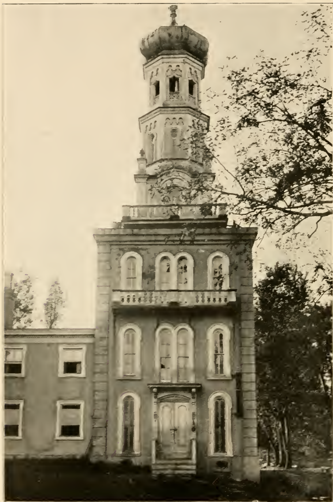
TOWER OF FISHER MANSION, REMOVED BY FILTER PLANT.
