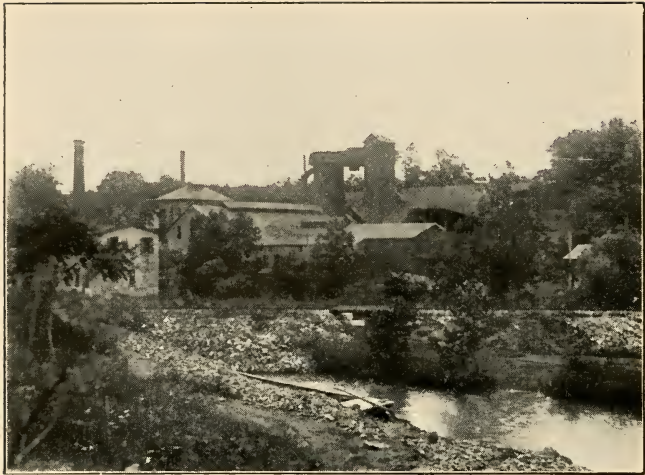
HISTORIC DURHAM FURNACE.
