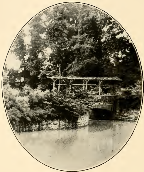
RUSTIC BRIDGE ON LINCOLN DRIVE.
