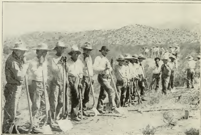
TRUCKEE-CARSON PROJECT, NEVADA
