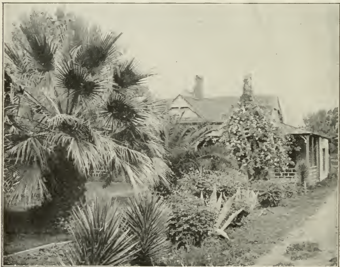
BUILDING HOMES IN ANTICIPATION OF THE OPENING OF GOVERNMENT WORKS ARIZONA
