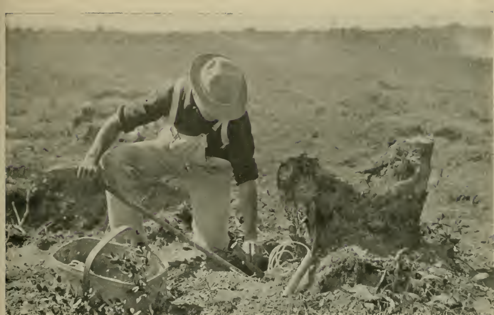
Placing one-half a pound of dynamite
