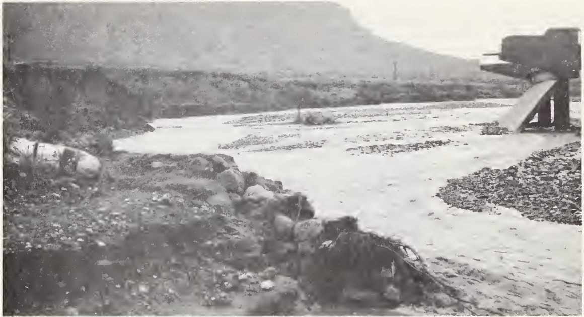
Bridge Damage Bridge on Highway 54 spanning Sulfur Draw The south abutment was washed out in August 1966.
