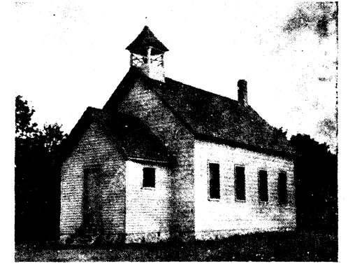
SCHOOL HOUSE, District No. 4, Banks Township.
