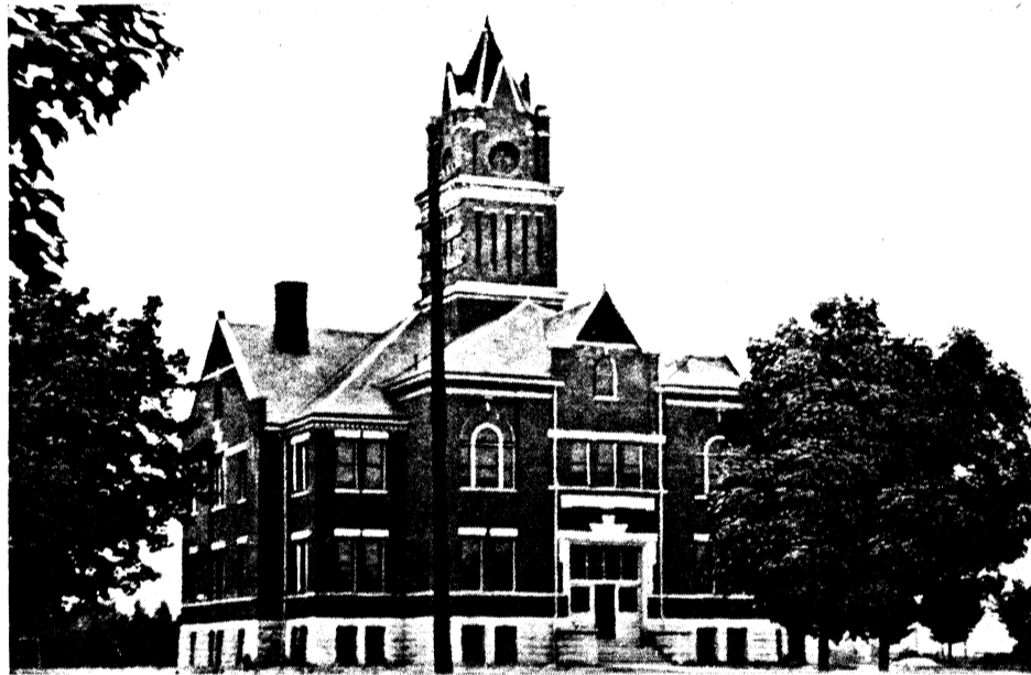
ANTRIM COUNTY COURT HOUSE, BELLAIRE, MICHIGAN.
