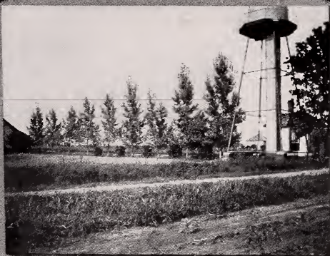
CAROLINA POPLARS SIX YEARS PLANTED. HEIGHT TO BOTTOM OF TANK 43 FEET
