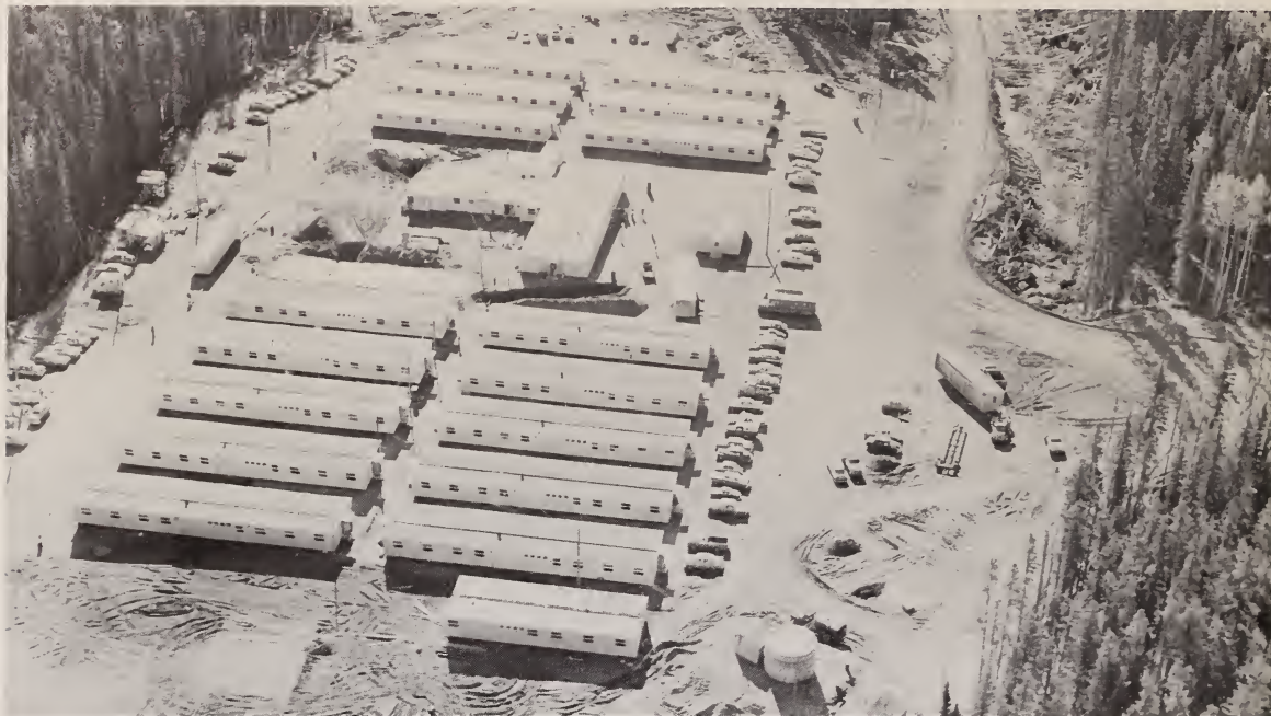
The construction camp at the Peace River division project, typical of a Canus-Prebuilt Co. Ltd. camp. One of the bunkhouse units is shown at right being moved into position, while the multi-unit group in the centre is the kitchen-dining building.
