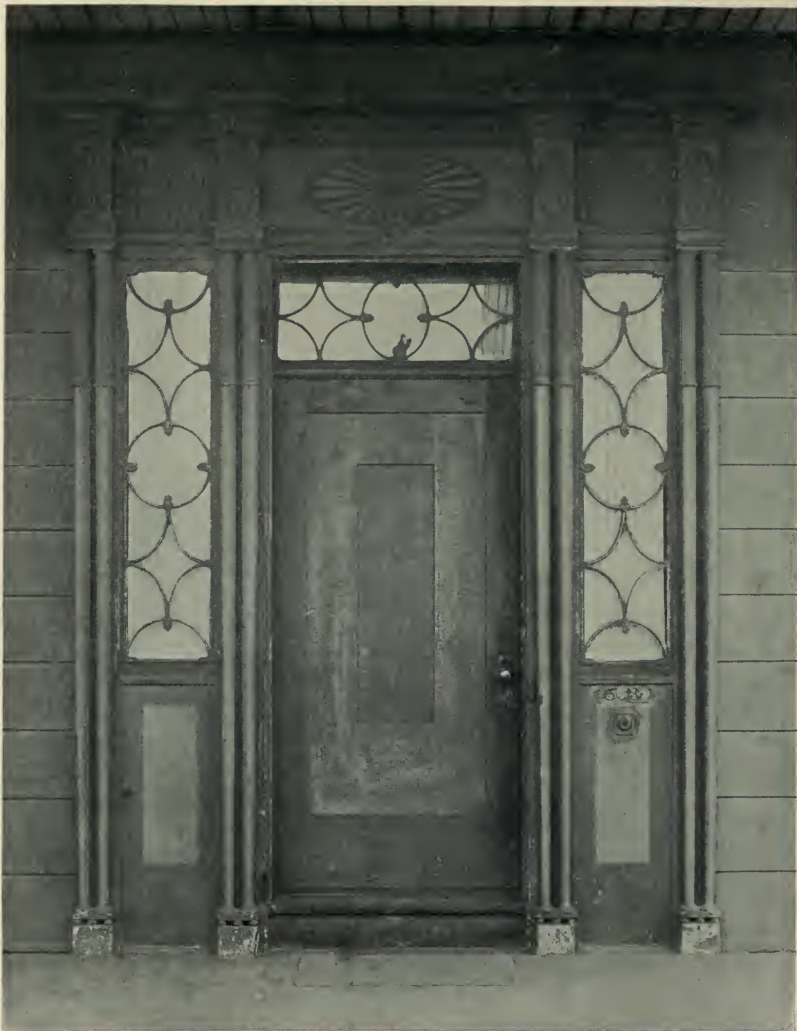
THE DOORWAY OF THE LEFFERTS HOUSE ON FLATBUSH AVENUE, FLATBUSH, L. I. Built in the 17th century, rebuilt about 1780
