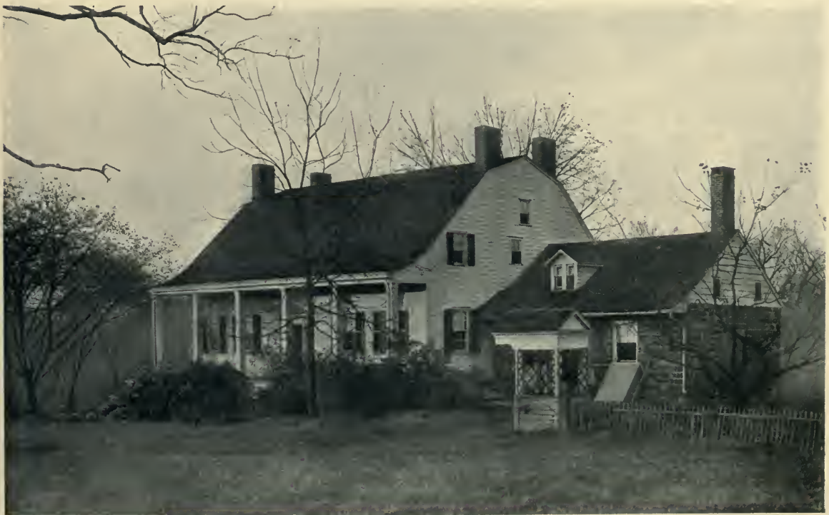
THE VREELAND HOUSE AT NORDHOFF, NEW JERSEY
