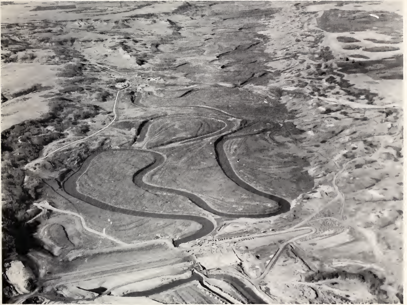
The Battle River project of Canadian Utilities, Limited, eleven miles southwest of Forestburg. The spillway is in the center foreground, while the initial construction of the plant building and pump-house can be seen up-stream. The valley which will contain the 1956 spring run-off can be plainly seen directly above the spillway. This picture was taken from an aircraft in the latter part of October 1955.
