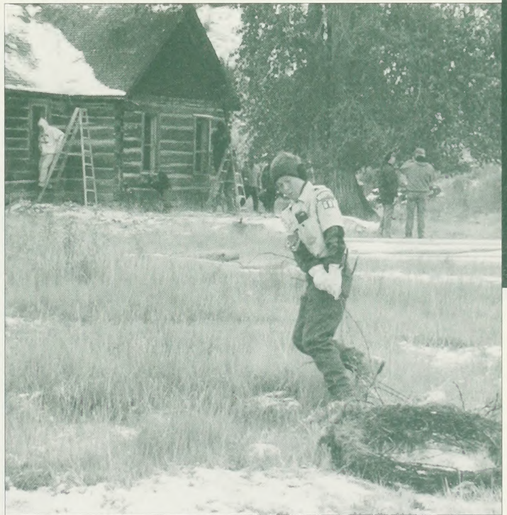
More than 60 National Public Lands Day volunteers helped with many projects at the Beaverhead River site near Dillon, Montana. Boy Scouts hauled away brush and debris, while other volunteers cleaned and bird-proofed the homestead cabin, which dates from the 1880s.
