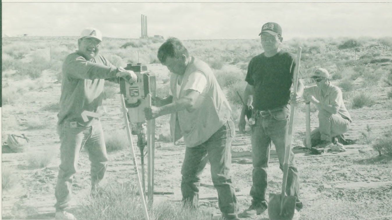
The BLM Cadastral Survey Program provides on-the-ground surveys to establish Federal and Tribal land boundaries. These legal boundaries provide for better management of valuable trust assets near the Navajo Nation Coal Power Plant.
