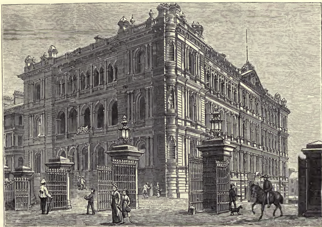
GOVERNMENT BUILDINGS, MACQUARIE STREET, SYDNEY.
