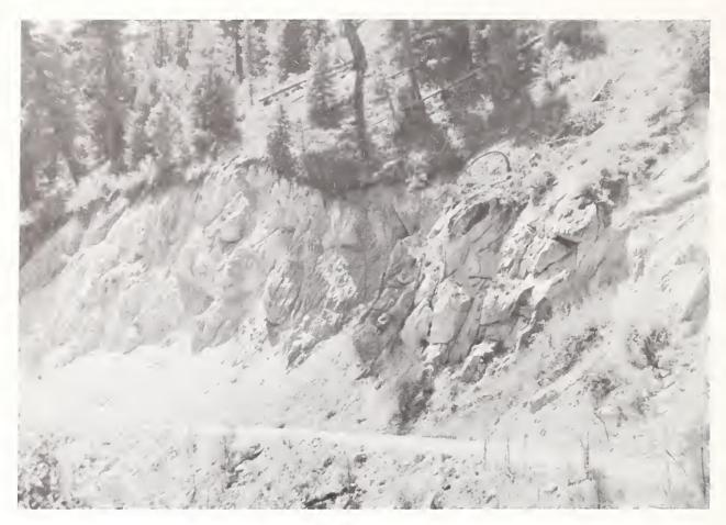
Figure 7.--Granitic rocks in the Idaho Batholith exhibit various degrees of weathering. Road cuts in the more highly weathered types continue to supply sediment for years.
