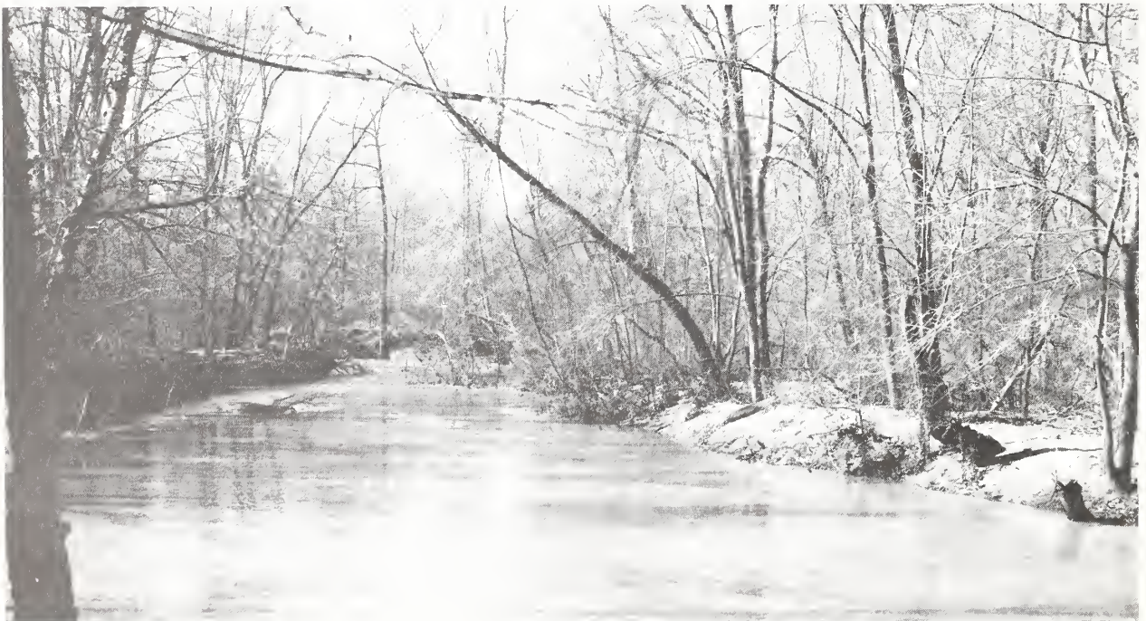
LITTLE BLACK RIVER IN ARKANSAS BELOW JUNCTION OF STATE LINE DITCH. NOTE BRUSH AND SAND DEPOSITED DURING FLOOD FLOWS. THIS DAMAGE WILL BE SIGNIFICANTLY REDUCED BY FLOODWATER RETARDING STRUCTURES AND INLET STRUCTURES ASSOCIATED WITH DRAINAGE DITCHES.
