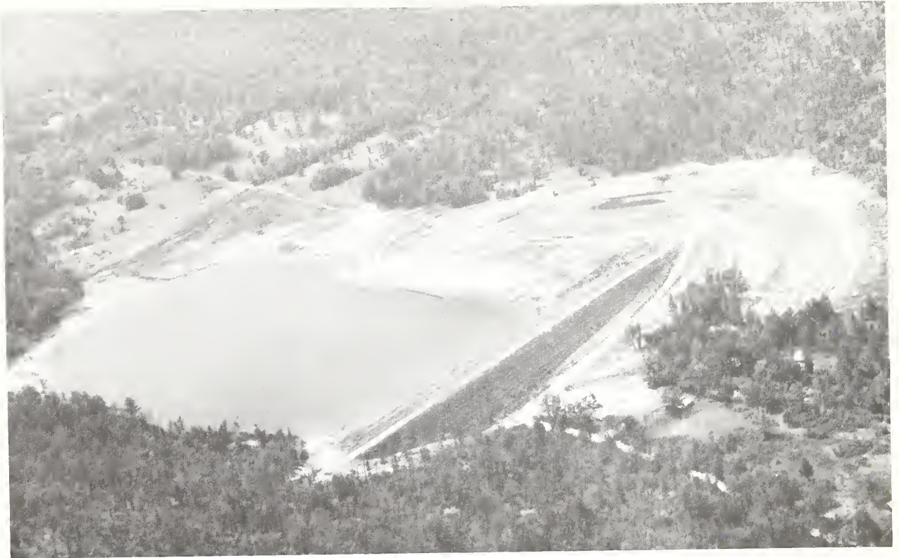
A CONSTRUCTED FLOODWATER RETARDING STRUCTURE IN ARKANSAS IN TOPOGRAPHY SIMILAR TO LITTLE BLACK WATERSHED.
