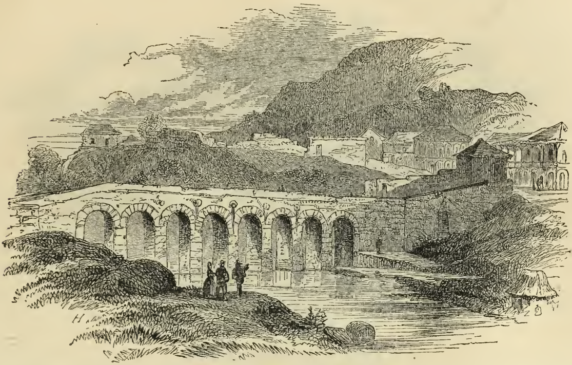
BRIDGE OF JUTECALPA.
