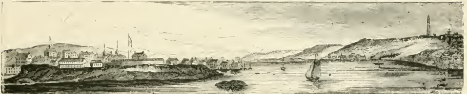
NEW LONDON HARBOR, NORTH VIEW.
