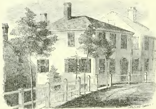
SITE OF THE COMMON HOUSE.
