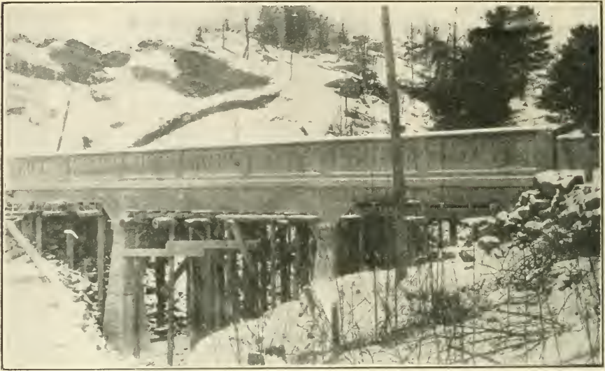
Little Kashee Bridge, Muskoka Road. Concrete Trestle, 78 feet long.
