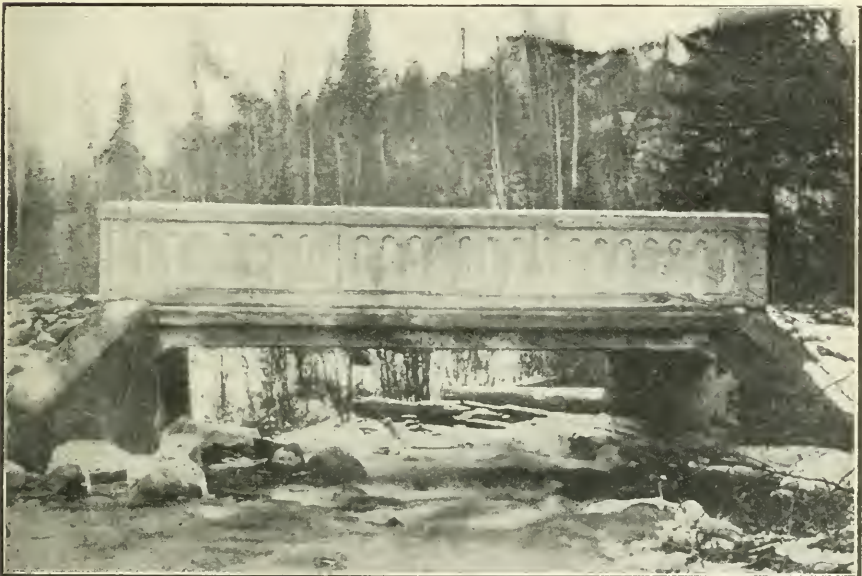
Spark's Creek Bridge, Bonfield. 20-foot Concrete Beam.
