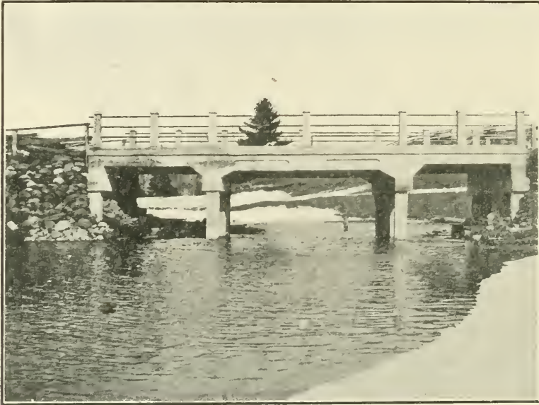
Hobart Bridge, Con. 7, Medonte. Concrete Pile Trestle, 43 feet long.
