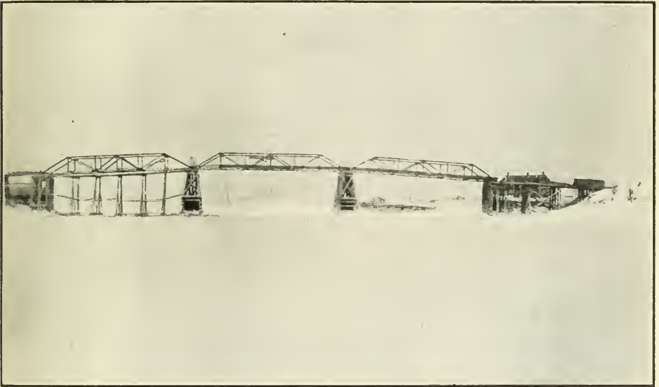
Judge Bridge, White River. Steel Spans on Timber Piers.
