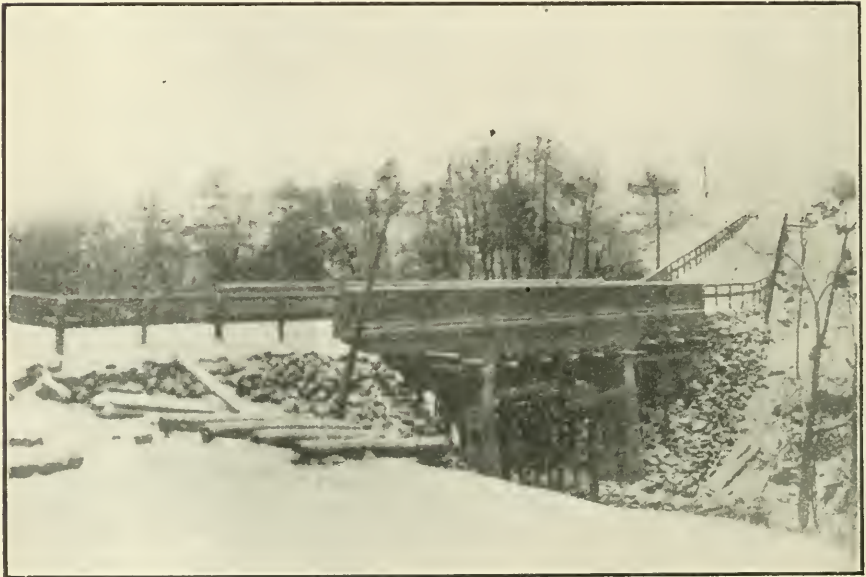
Little Kashee Bridge, Muskoka Road. Concrete Trestle, 78 feet long.
