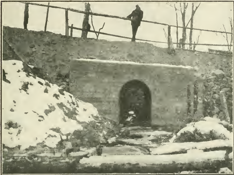
North Road Culvert, Algoma.
