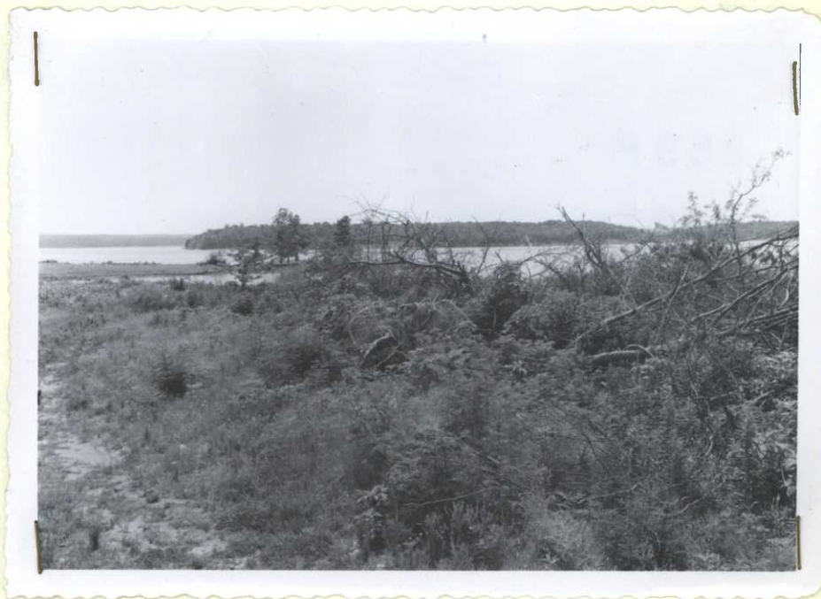
Dozed tree completely fill the old eroded roadbed at Sulphur Wells. Soil and Moisture Operations. CRM.
