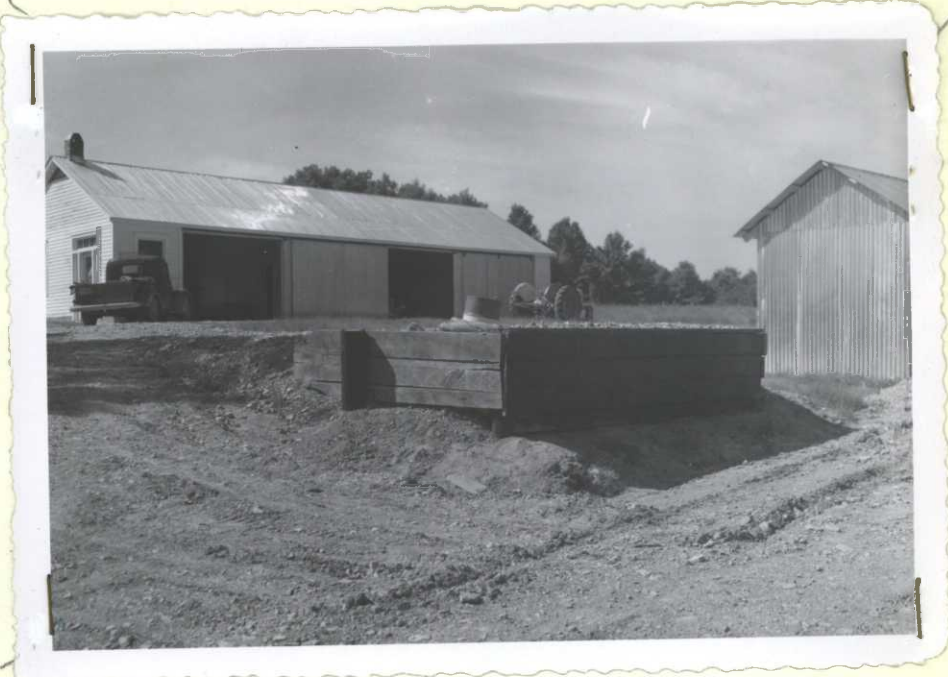
New loading ramp constructed at Big Sandy work center. CRM.
