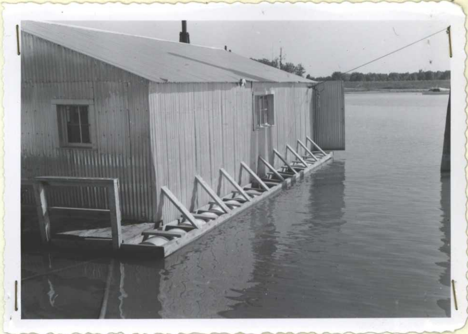
New out-rigger placed on floating boathouse at Paris Landing. CHG.
