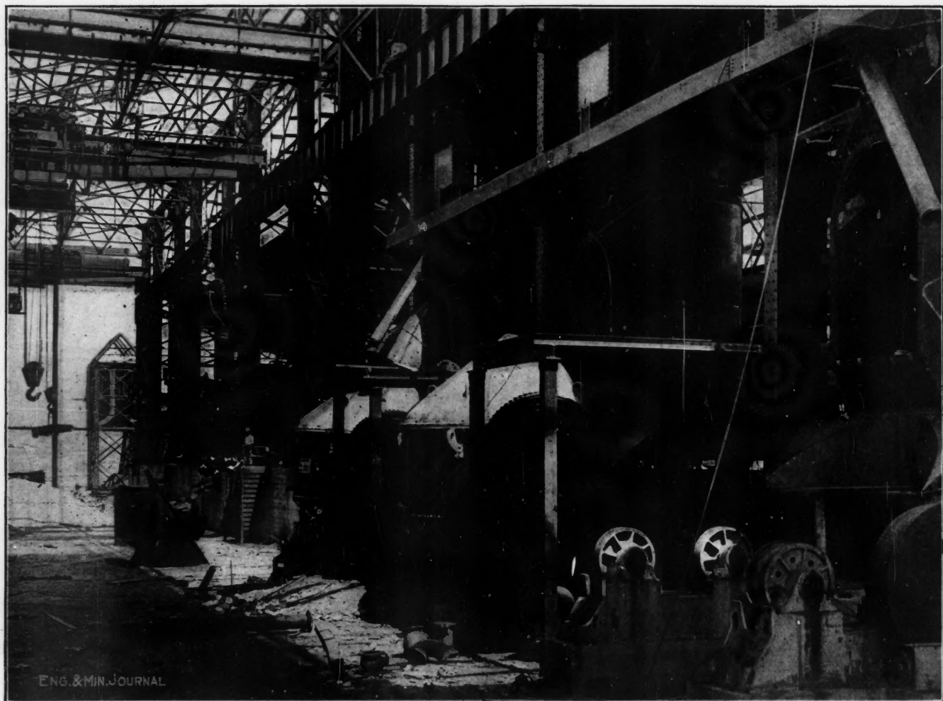
CONVERTER AISLE DURING CONSTRUCTION—AGGLOMERATING PLANT IN BACKGROUND
