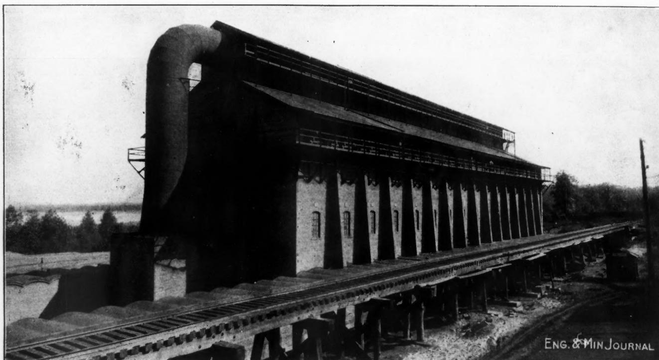
BAGHOUSE OF ST. JOSEPH LEAD CO.—LOOKING SOUTH
