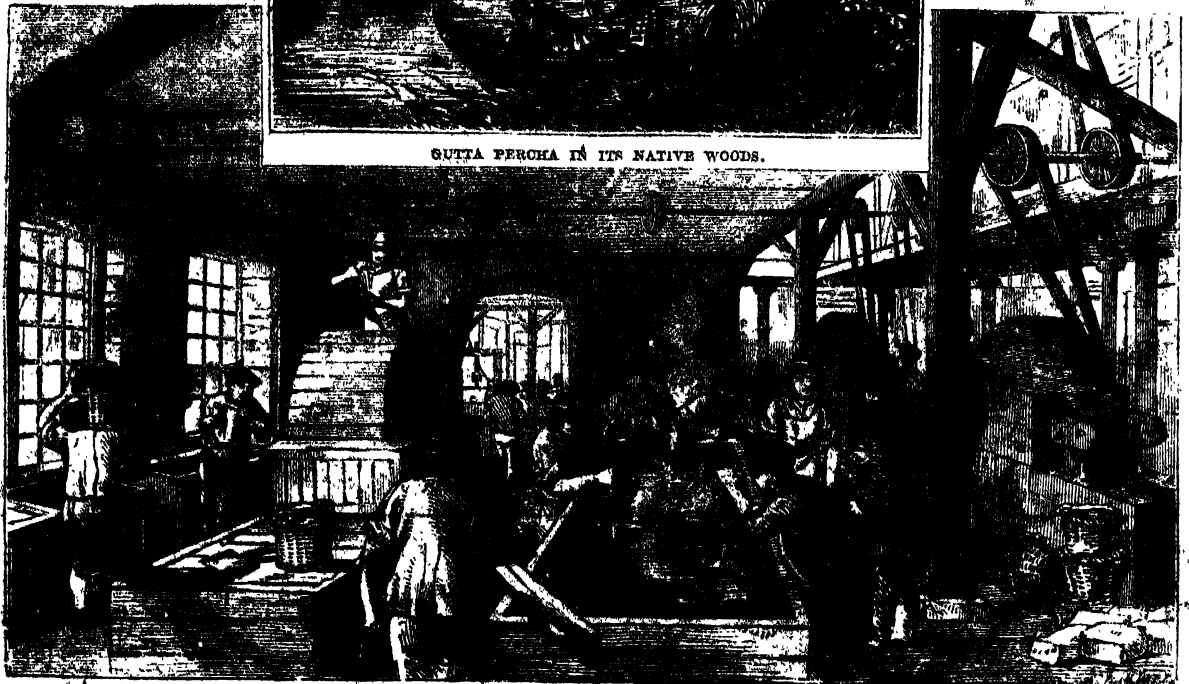
GUTTA PERCHA—ROLLING ROOM AND PRESS.
