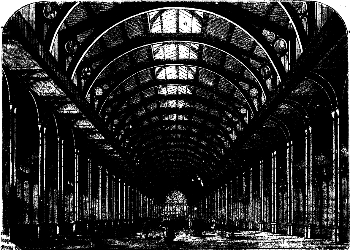
INTERIOR OF THE BUILDING.
