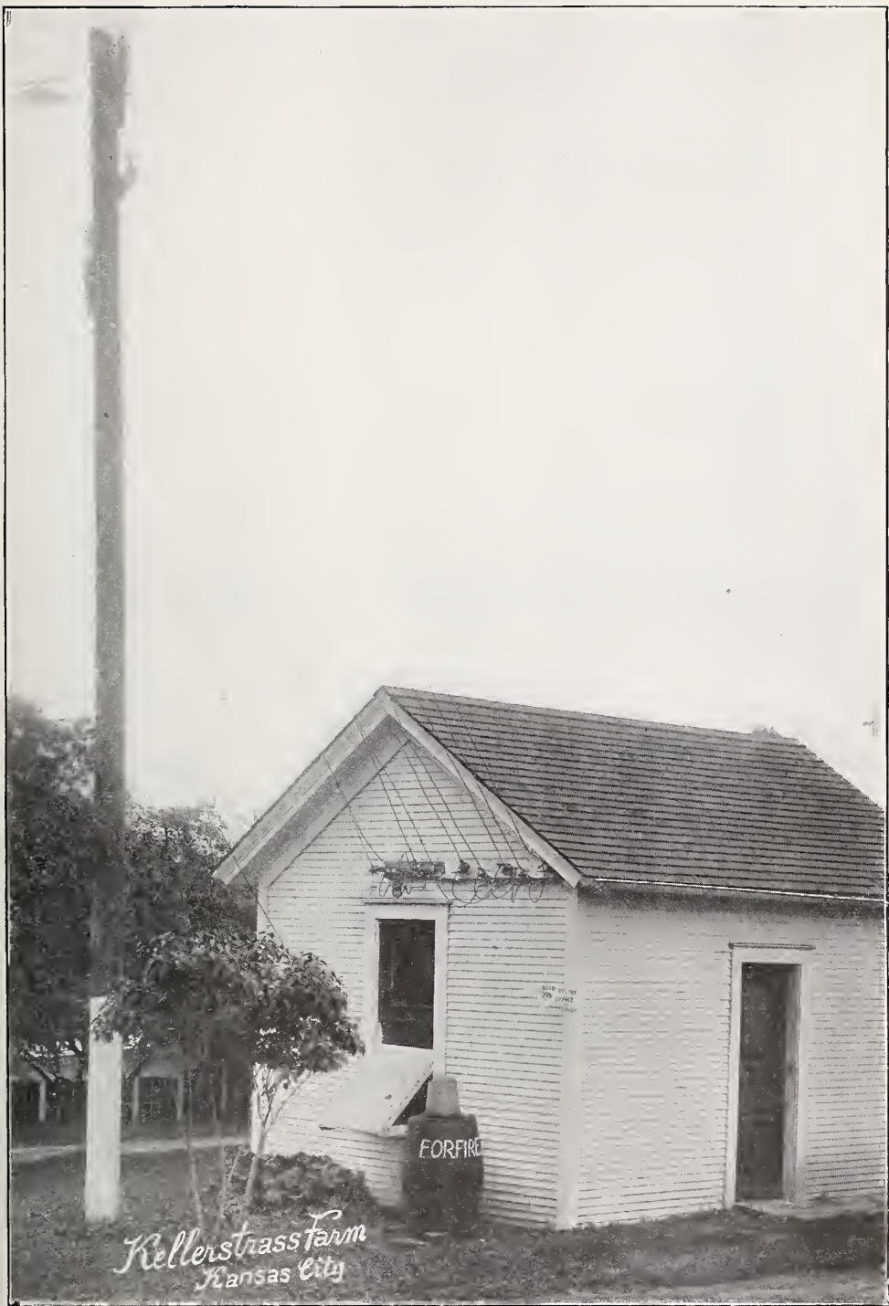
No. 44. Electric light plant on the Kellerstrass Farm
