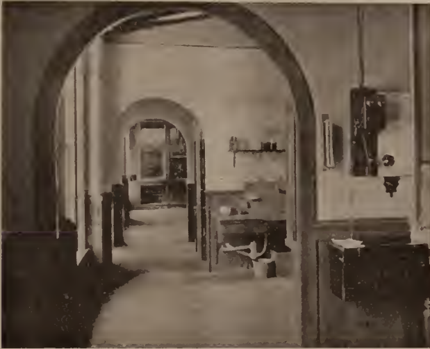
CORRIDOR CONNECTING FOUR OF THE WORKING ROOMS.
