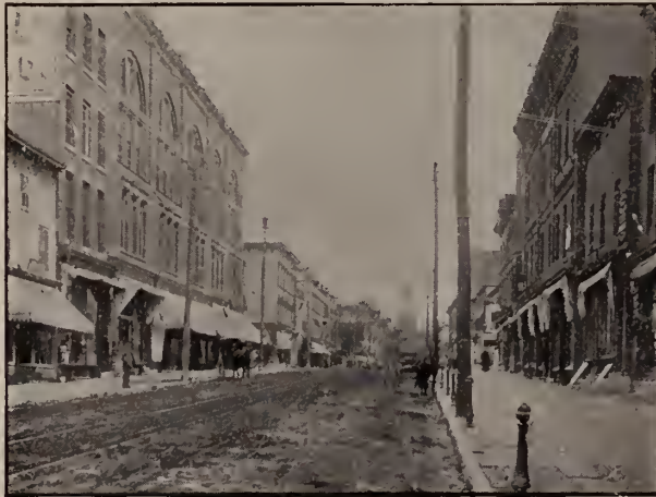
CHURCH STREET—LOOKING NORTH.
