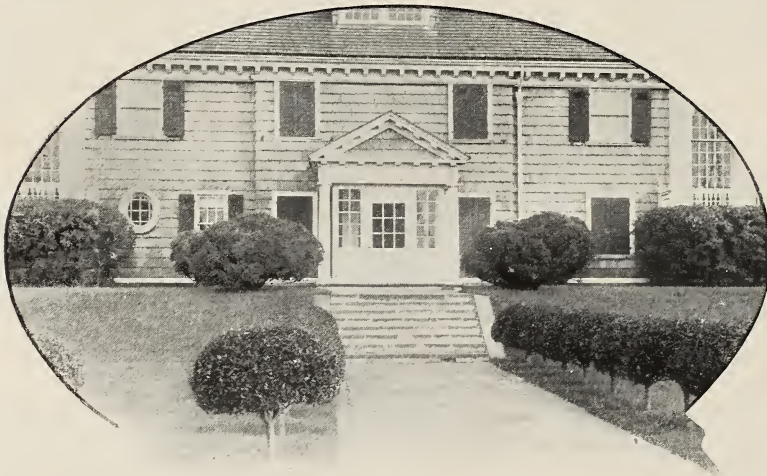
The large dwarf Boxwood trees flanking the entrance were moved by our Evergreen Tree-Mover, and are very old. The rows of Standard Privet on either side of the path are in keeping with the general scheme of decoration. "Wheatlands," the residence of Mr. E. D. Morgan.
