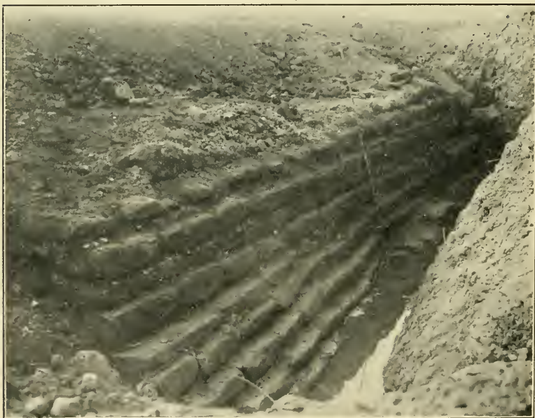
Fig. 13.—The dwelling-house: offsets at north corner.
