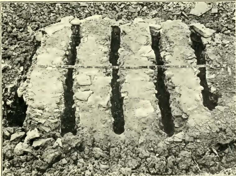
Fig. 27.—The round pottery kiln: the cross-walls, showing material used in construction, and cross flues. To face p. 38.
