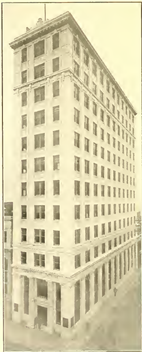
COMMERCIAL NATIONAL BANK BUILDING
