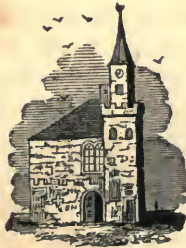
PARISH CHURCH—OLD TOWER AND SPIRE.
