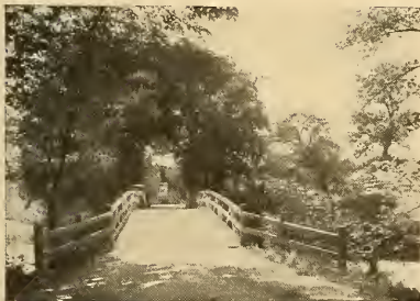
Concord Bridge. No. 176
