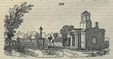
the summit of the cupola of this house there was originally a lamp with three burners and three separate reflectors. Two of the reflectors directed the light along the road in opposite directions, to show what might be coming or departing on either hand; the third reflector threw the light directly across the road, and down on the gate, for the purposes
