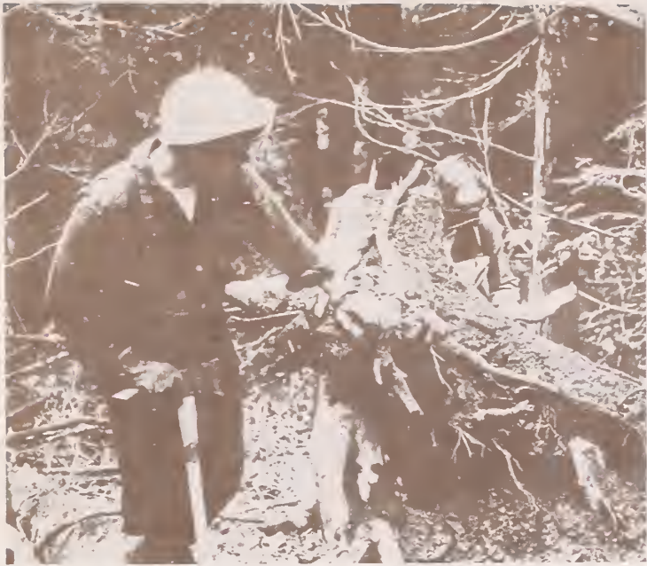
Figure 16. Blasting breaks rotted roots; the sound ones remain intact. University of Idaho, 11.
