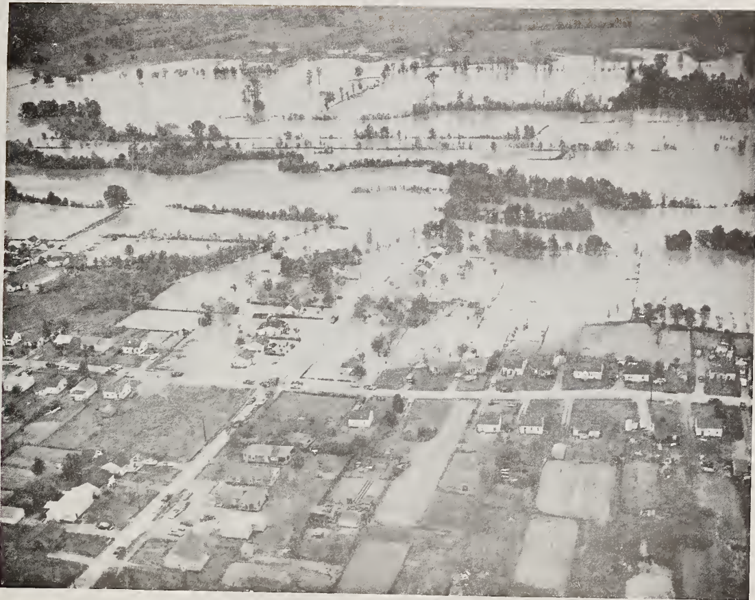
Photo 3 - May 9, 1958 Flood - Corner Watson and Barr Streets
