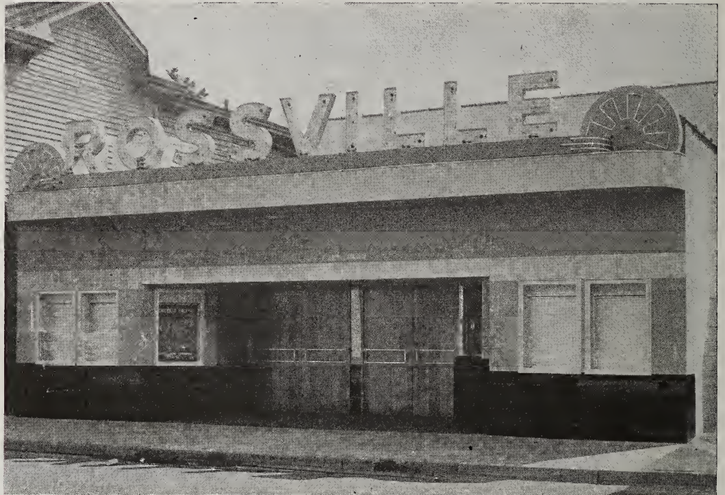
The marquee-less front of the Rossville has a protective ledge over a set-back entrance.
