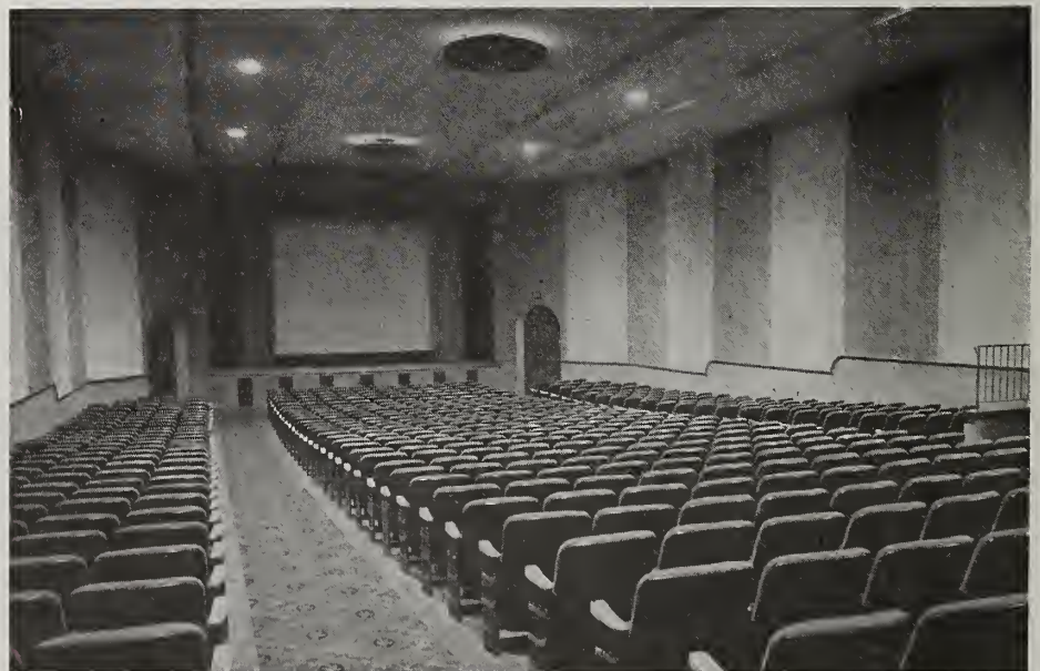
The auditorium has side walls with panels alternately of acoustic and hard plaster.
