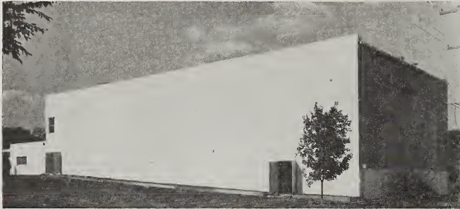
Completed side wall, with Vercalite slab bolted to steel frame.
