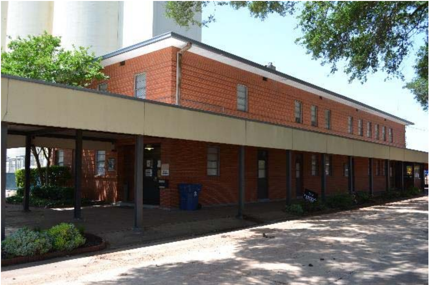
Photo 19 - Engineering Building (Resource ID 2), south and east elevations, view northwest
