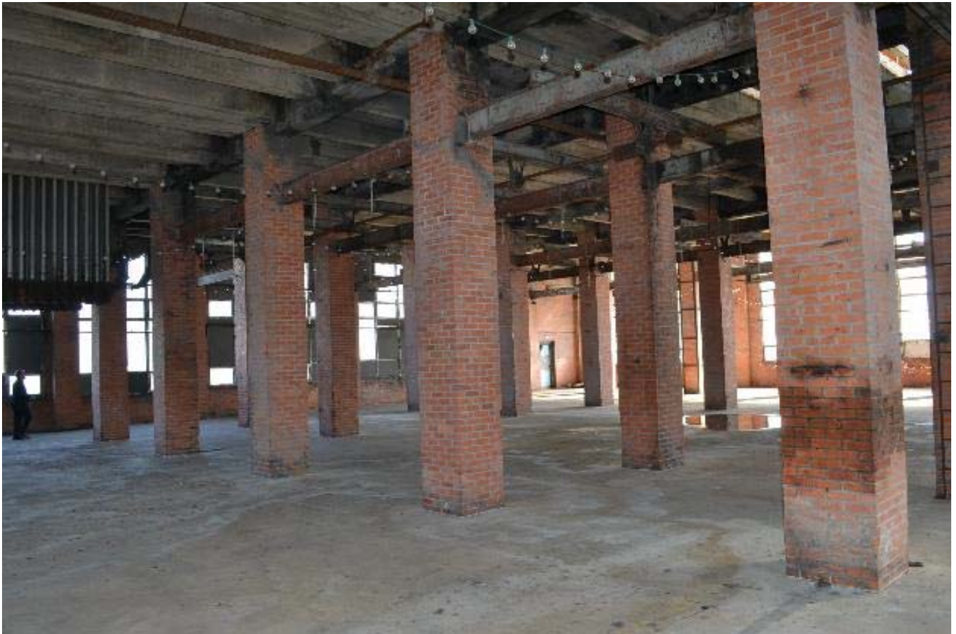
Photo 8 – Char House (Resource ID 1), interior, view northwest
