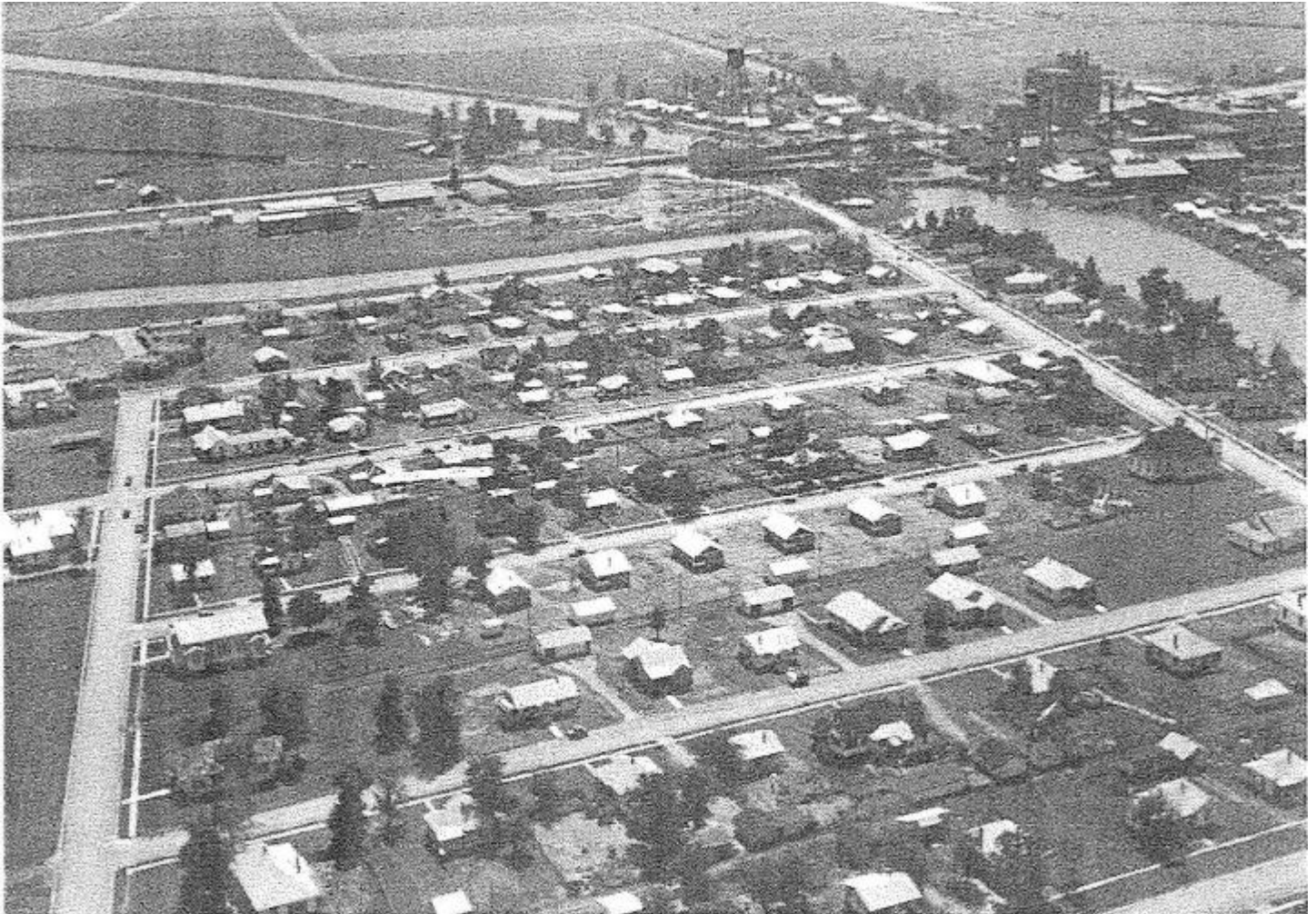
Figure 7 - Aerial of Sugar Land, looking south c. 1926. Char House in upper right corner. Courtesy Sugar Land Heritage Foundation.
