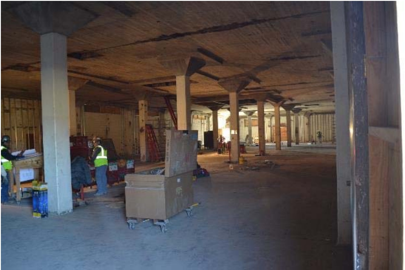
Photo 17 - Container Warehouse (Resource ID 5), interior, view west
