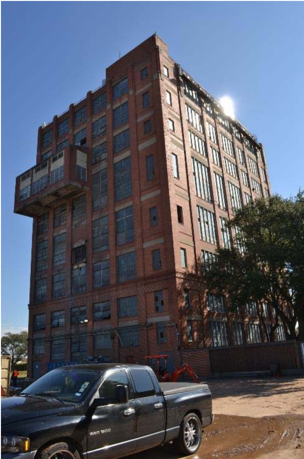
Photo 6 – Char House (Resource ID 1), north and west elevations, view southeast
