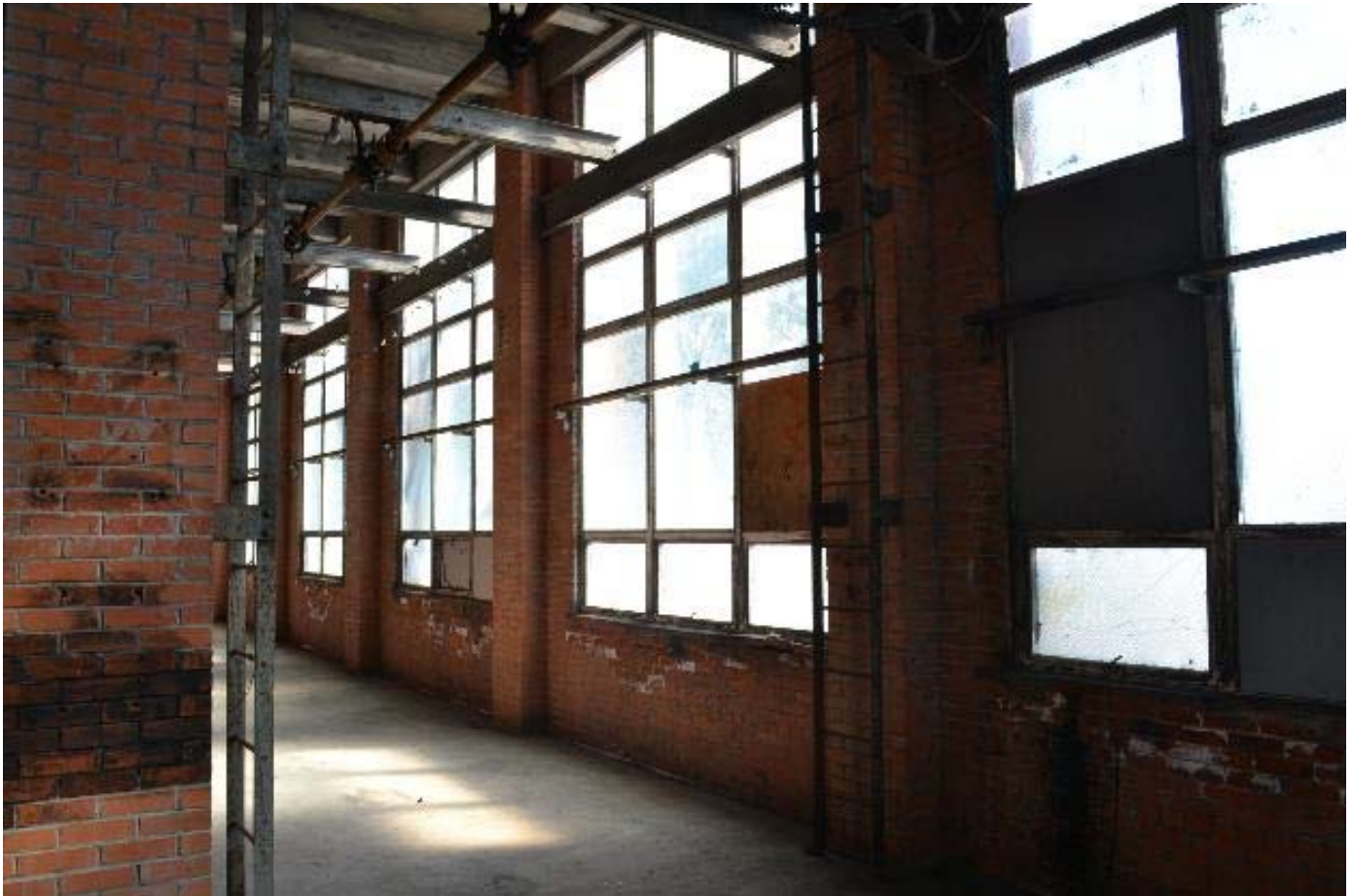
Photo 9 – Char House (Resource ID 1), interior, windows on the south elevation
