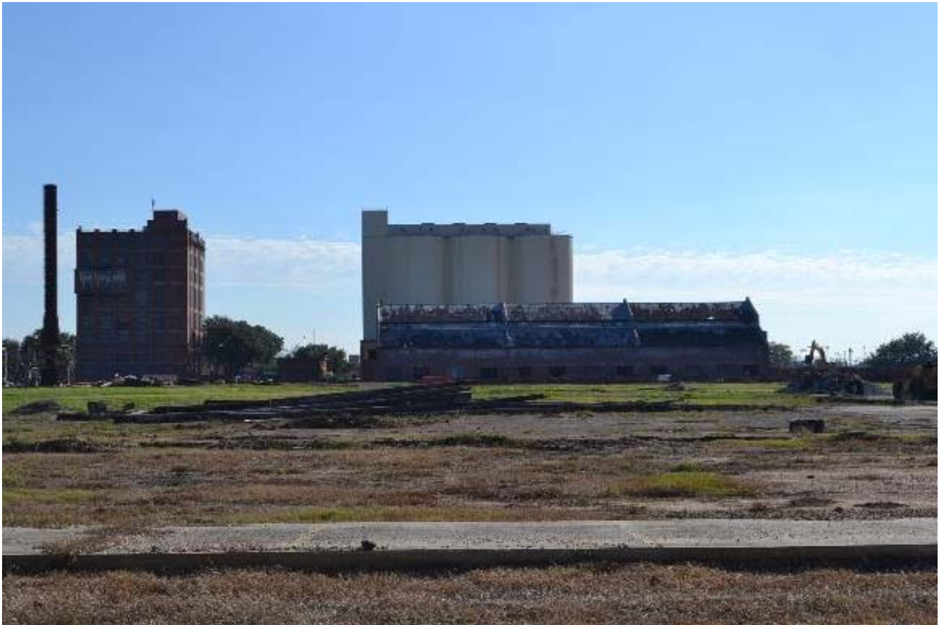
Photo 2 – Overall site, view south from north
