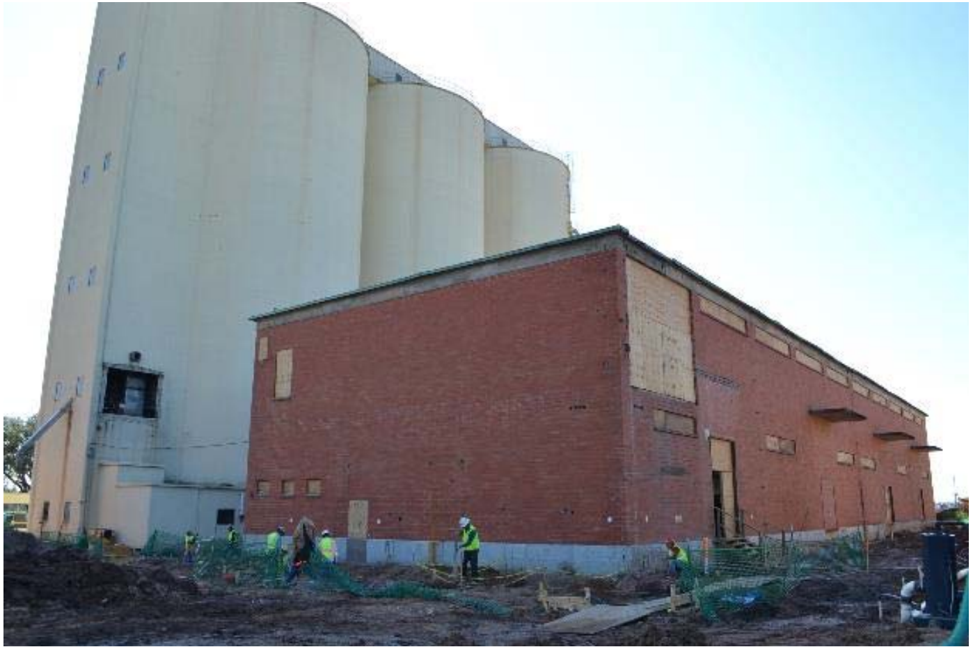
Photo 16 - Container Warehouse (Resource ID 5), east and north elevations, view southwest; silos (Resource ID 3) in background
