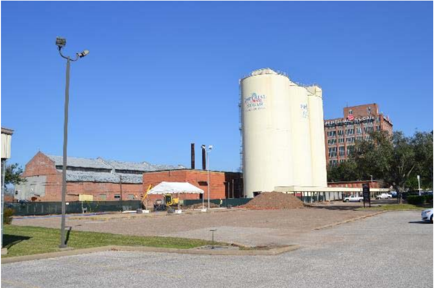
Photo 1 – Overall site, view northeast from west
