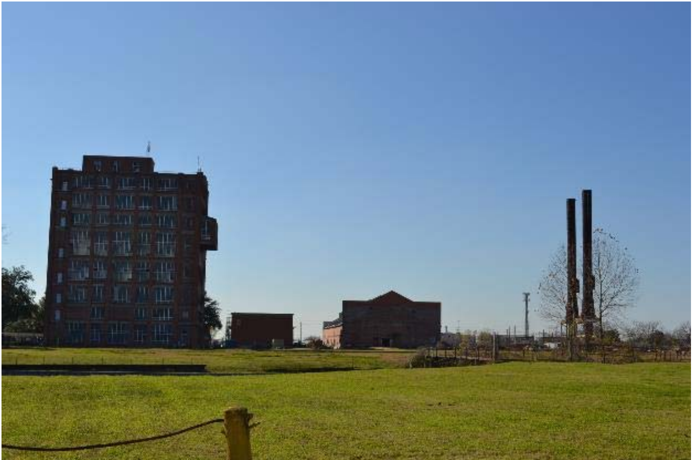
Photo 3 – Overall site, view west from east
