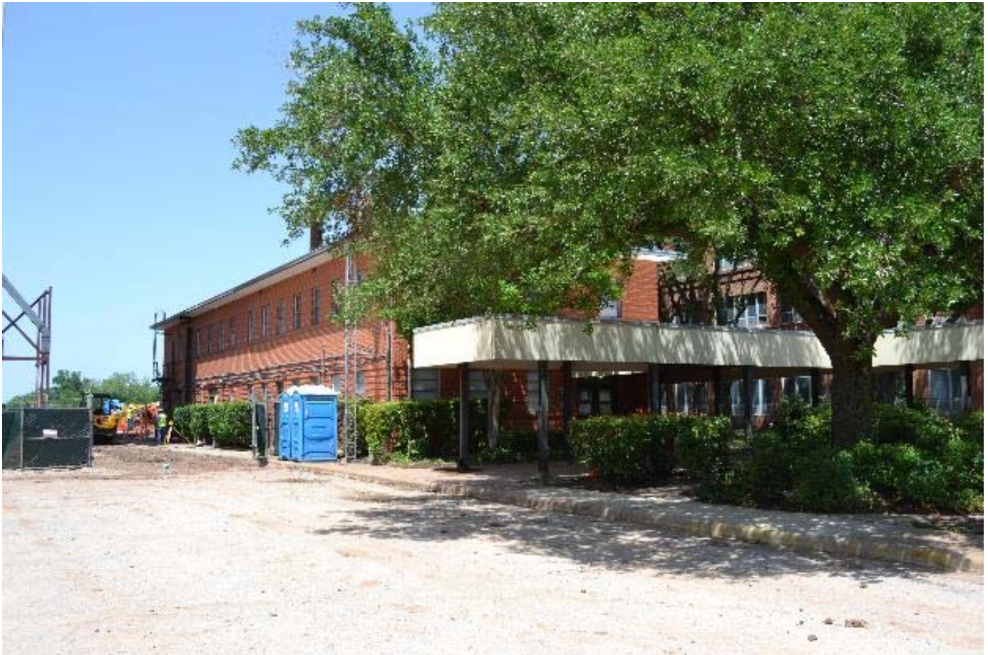
Photo 20 - Engineering Building (Resource ID 2), west and south elevations, view northeast
