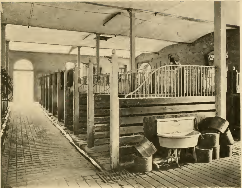
FIG. 130.—A model work horse stable, showing width of stalls, corrugated concrete floors, wooden racks in stall floors, width of alleys, drains and ventilating flues.
