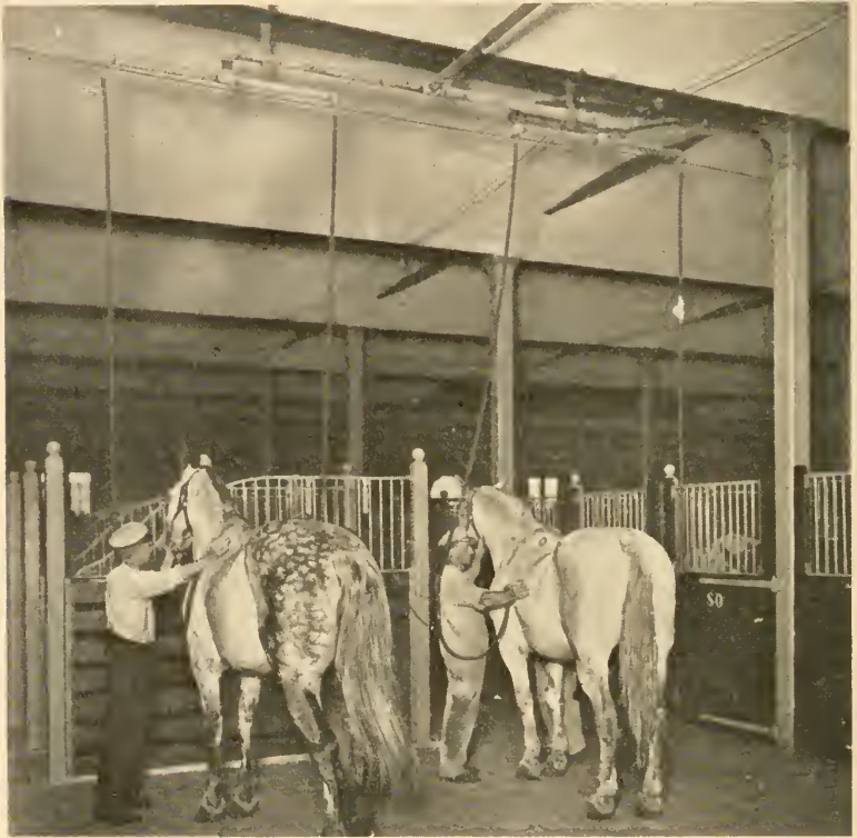
FIG. 134.—A vacuum grooming machine in operation. A vacuum is maintained in the pipes which draws the dirt out of the hair and conveys it to a receptacle where it collects and can be removed.
