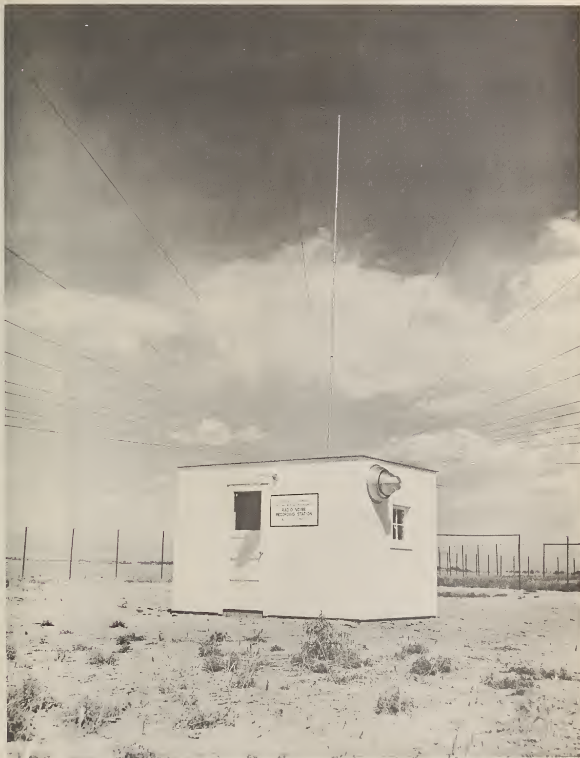
Radio Noise Recording Station
