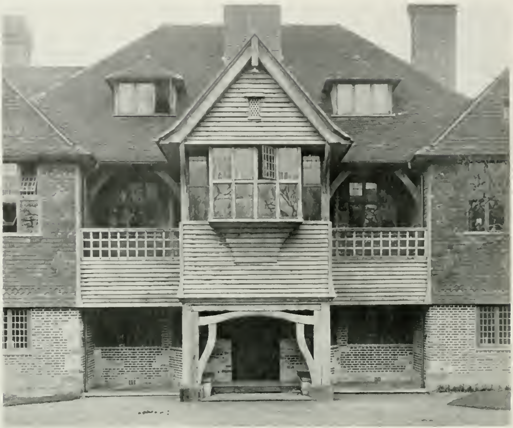
"SHOVELSTRODE MANOR," EAST GRINSTEAD : FRONT ENTRANCE PORCH.
