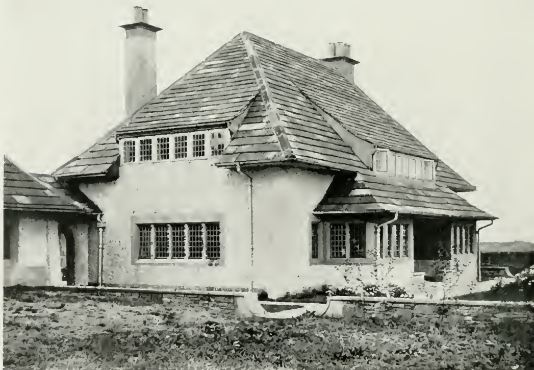
View from South-West.
