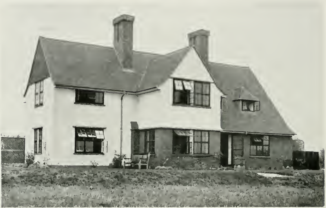
View from South-West.
