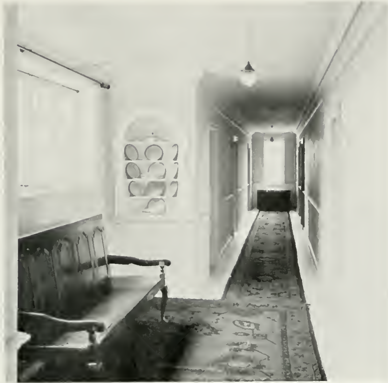
Corridor, First Floor.
