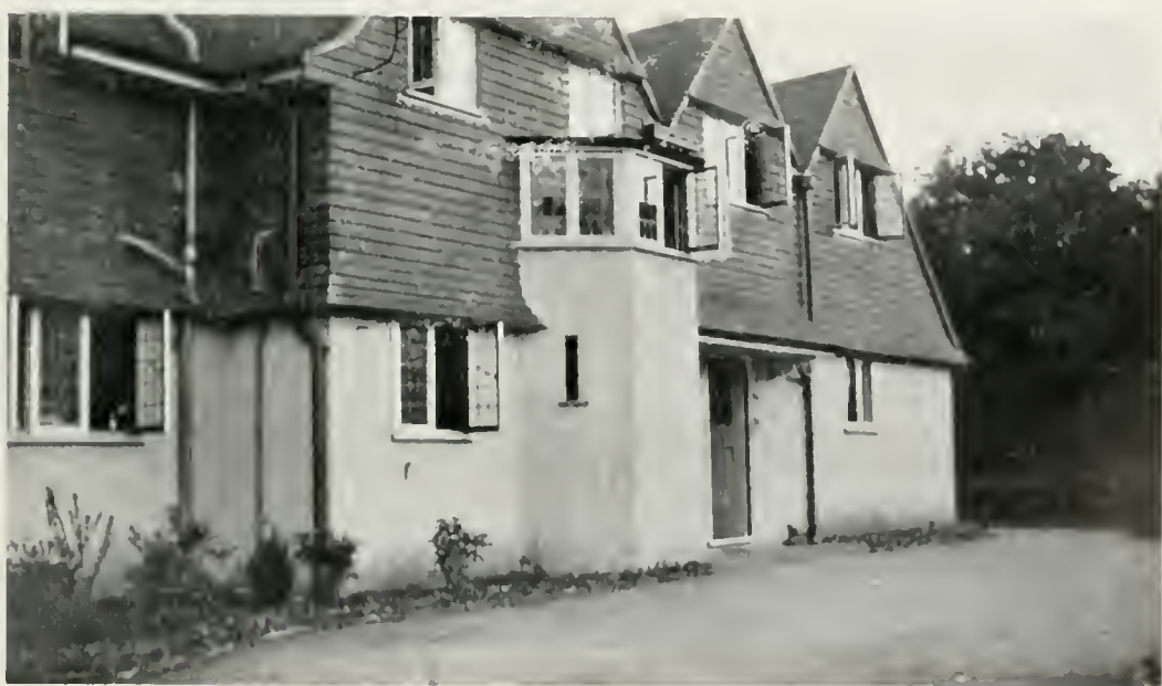
"BUNCH COTTAGE," HASLEMERE : DETAIL OF ENTRANCE FRONT.
