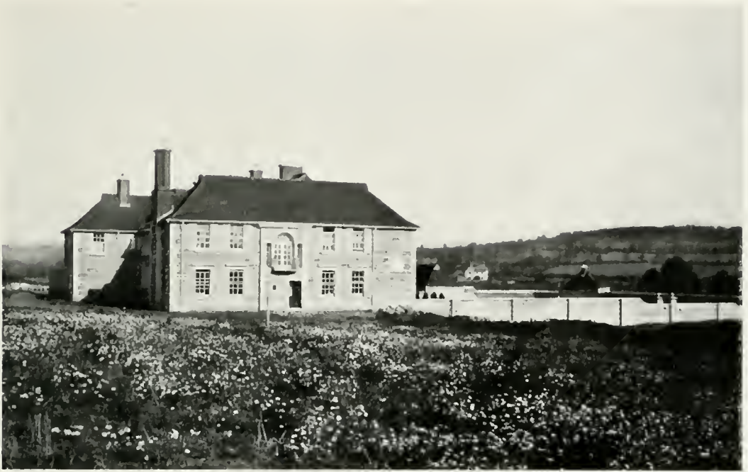
View from South-West.
