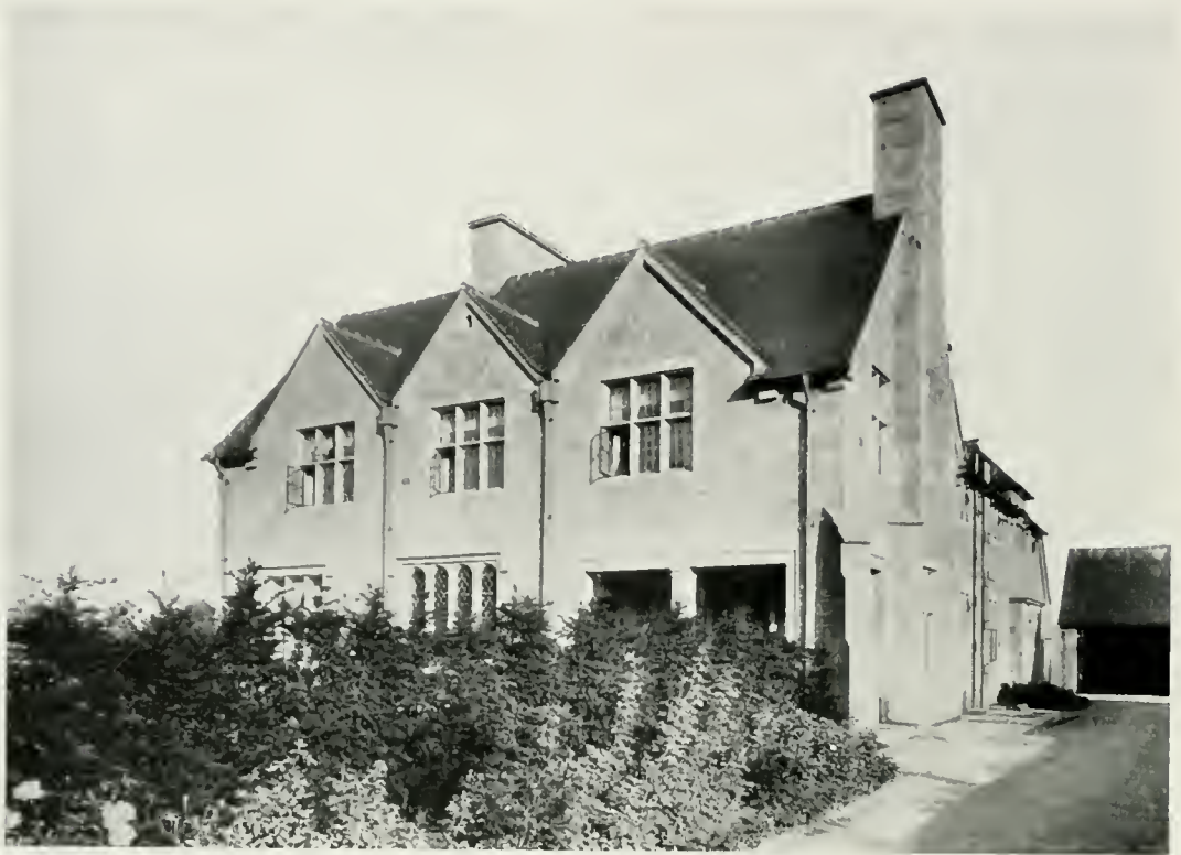
Exterior from Drive.
