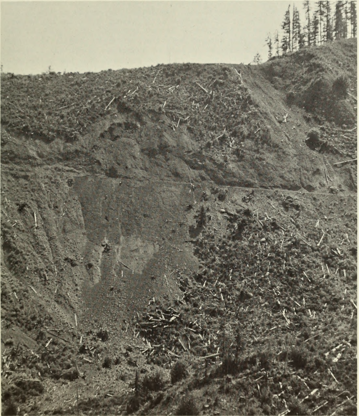
Figure 20 Loss of site productivity from erosion and dry ravel on extremely steep slopes of Digger (66) and Jason 64 soils in the Roseburg Formation. Deep cuts in very incompetent bedrock would have been eliminated by location of road along ridge-top.
