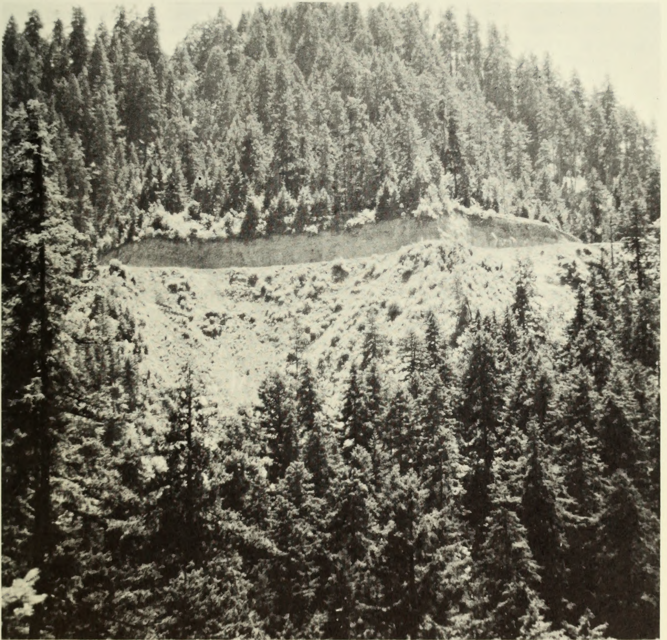
Figure 23 Debris avalanches initiated by the sidecast of waste materials from deep cuts during road construction in Digger (66) and Jason (64) soils.
