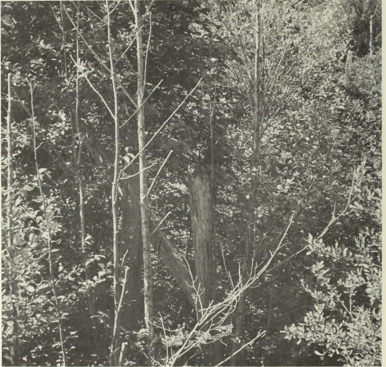
Figure 30 Fifty year old pilings of Port Orford Cedar used to provide support for old logging railroad trestles located in tributary drainage headwalls of Baker Creek along BLM access road in the Otter Point Formation.
