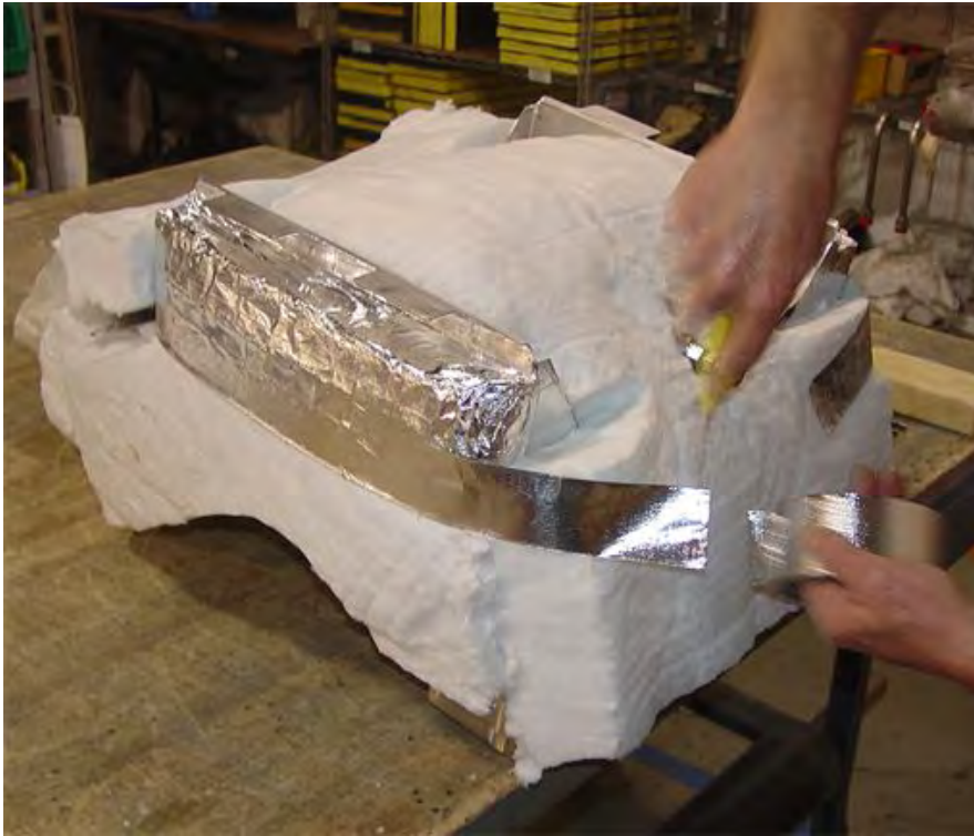
Figure 23. Trimming Insulation on the Plenum (Sheet 2 of 2).
