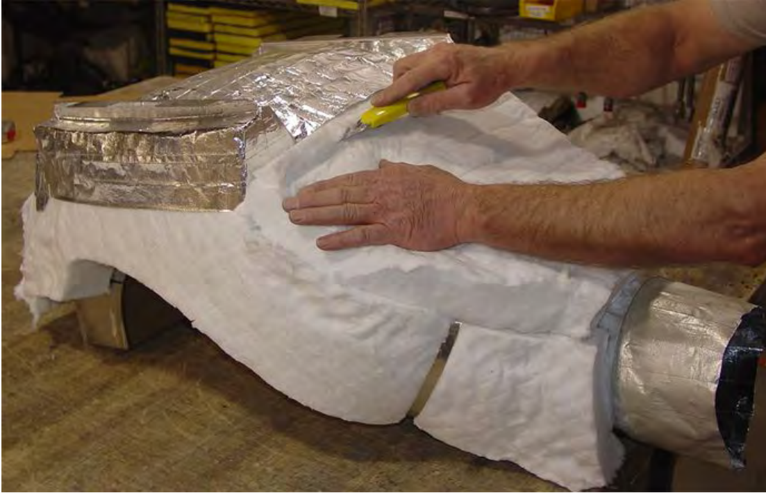
Figure 26. Trimming Insulation from Plenum (Sheet 2 of 2).
