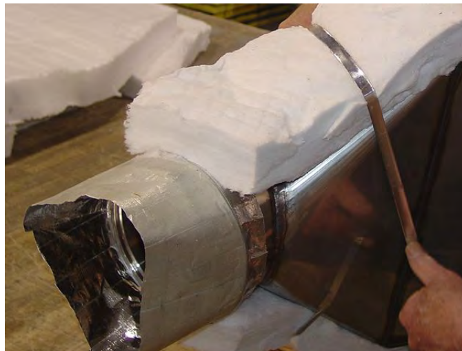
Figure 20. Preparing Insulation for Taping (Sheet 2 of 2).
