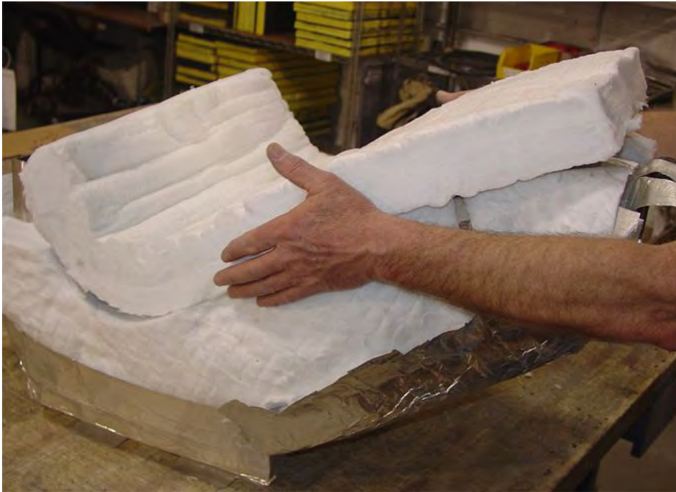
Figure 30. Snugging Insulation into the Bend (Sheet 1 of 2).
