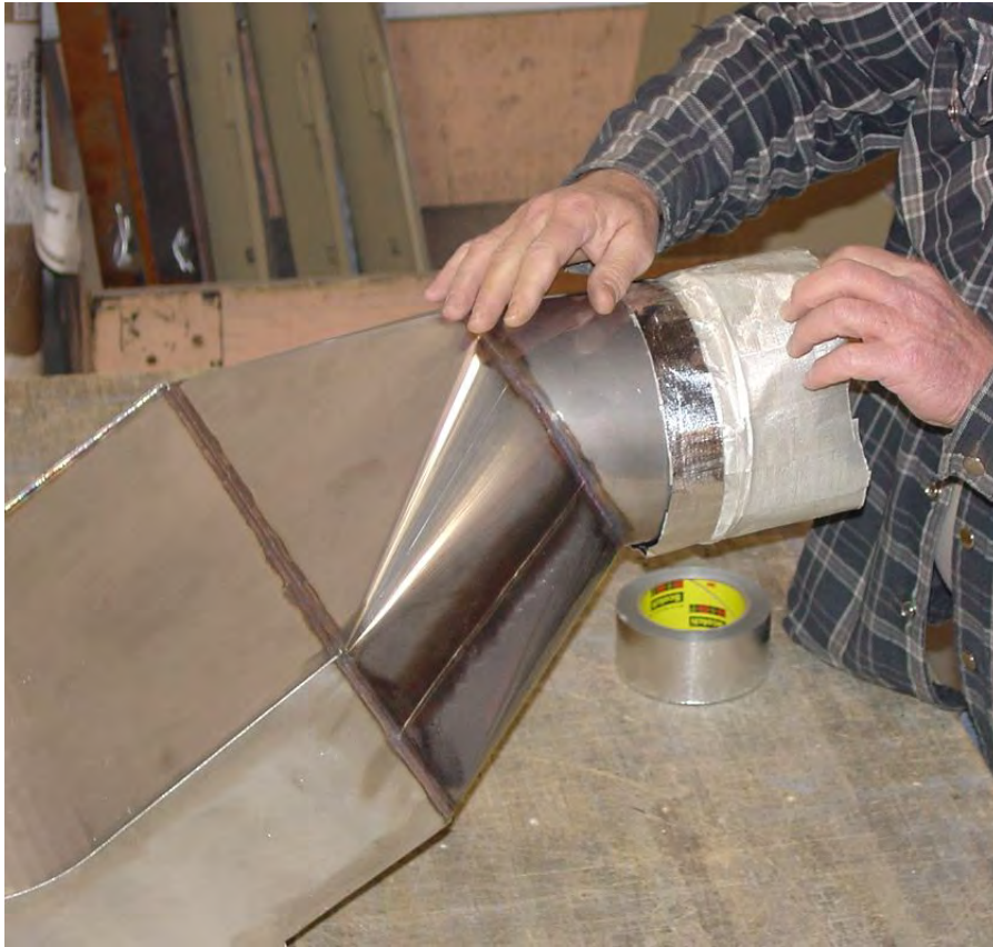
Figure 16. Inlet Taping.
