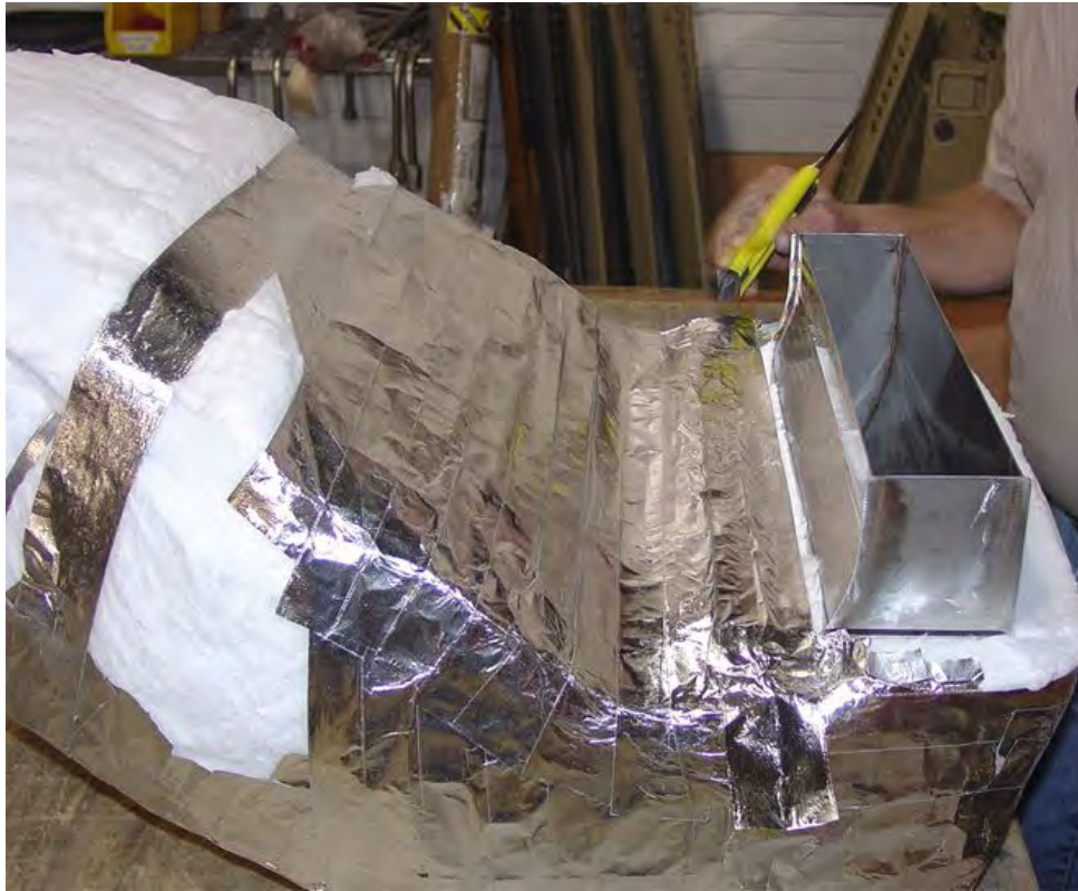
Figure 35. Building the Nonstick Side Around the Plenum Outlet.
