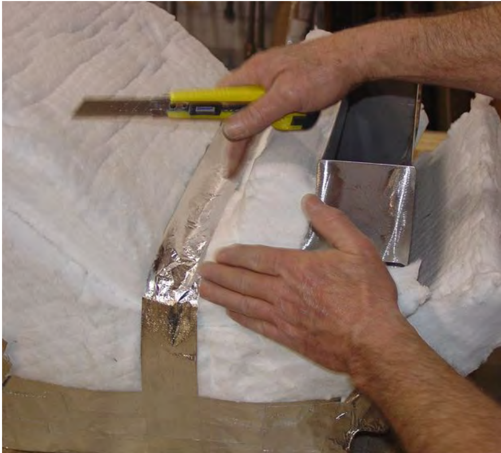
Figure 31. Taping Bend to Keep it in Place (Sheet 1 of 2).
