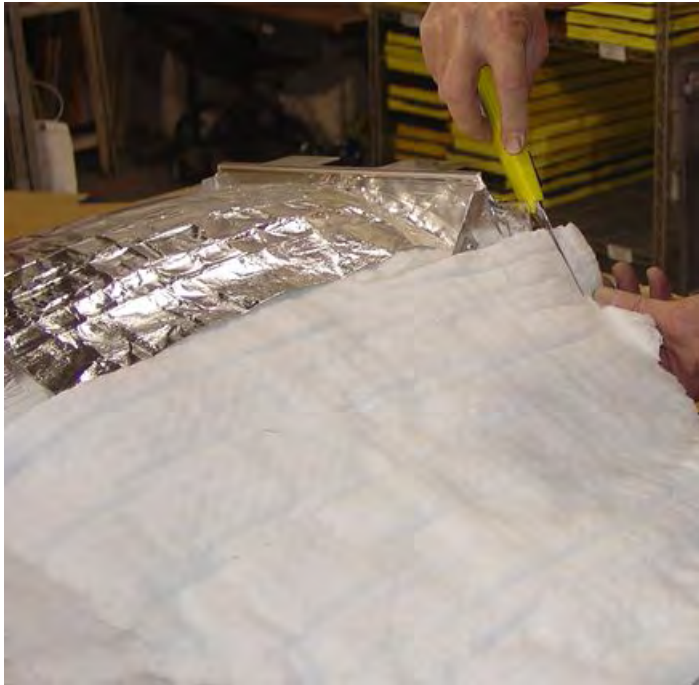
Figure 27. Trimming Insulation Around the Inlet (Sheet 1 of 2).
