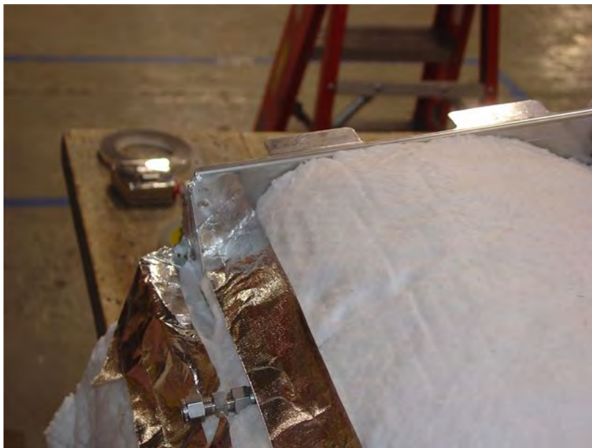
Figure 24. Taping Down the Insulation (Sheet 2 of 2).
