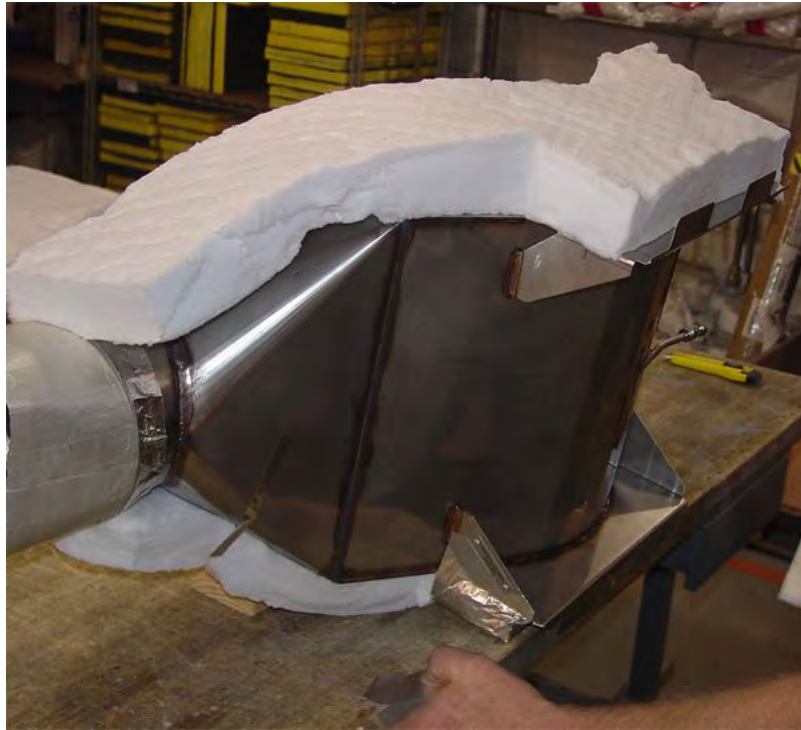
Figure 20. Preparing Insulation for Taping (Sheet 1 of 2).
