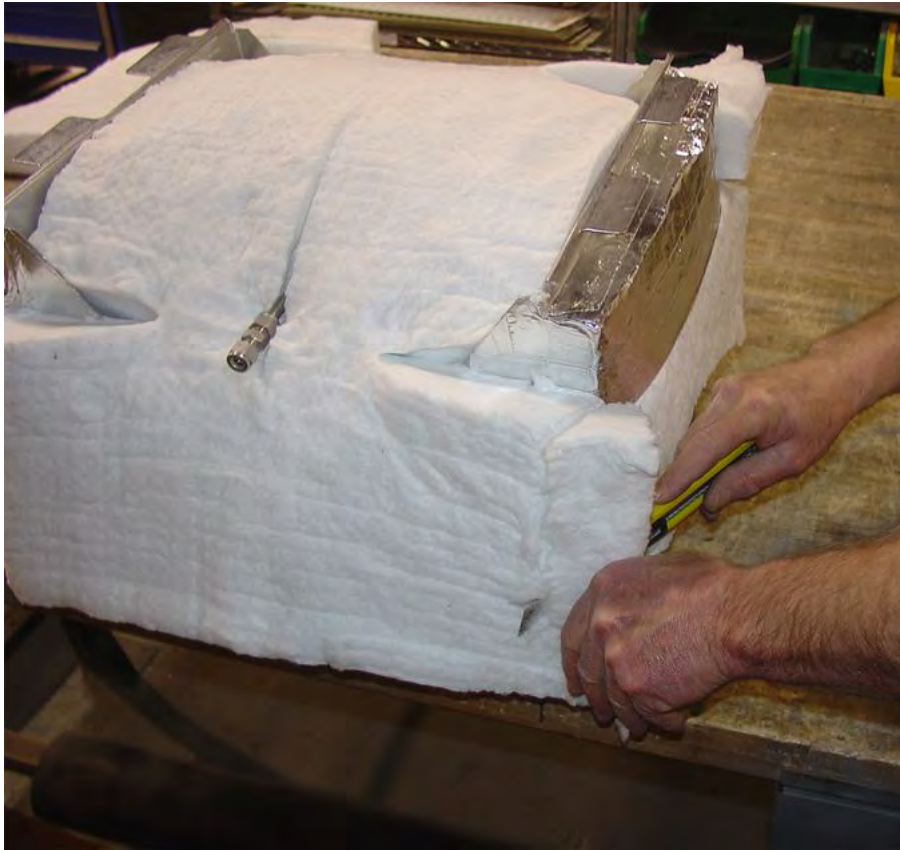
Figure 23. Trimming Insulation on the Plenum (Sheet 1 of 2).
