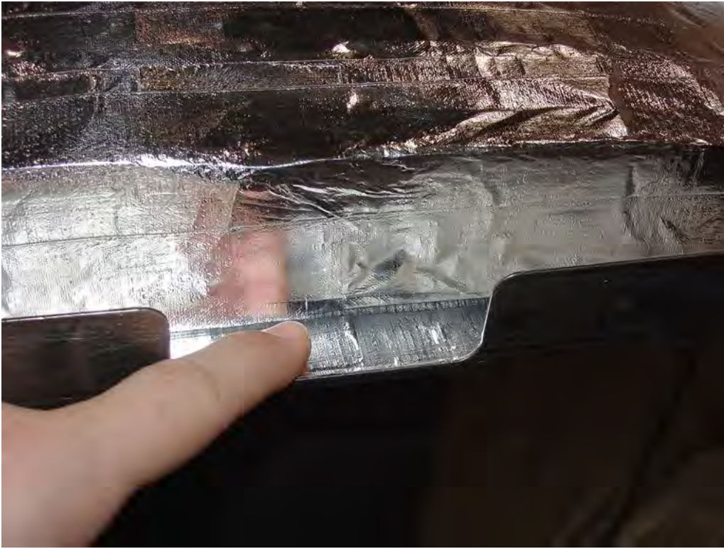
Figure 19. Taping of the Plenum (Bottom).
