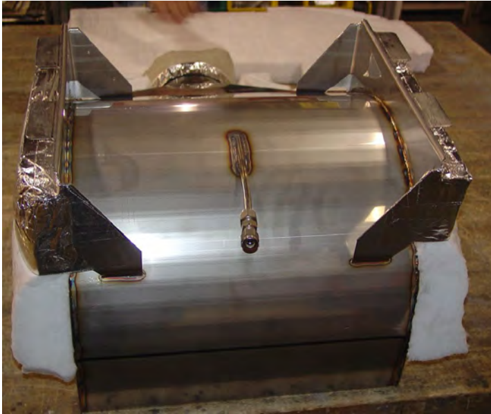
Figure 21. Placing Insulation on Bottom of the Plenum.
