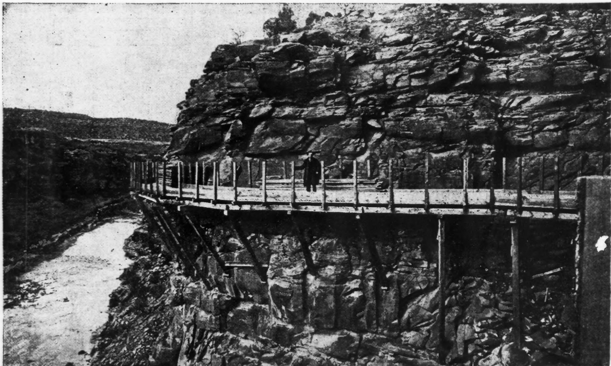
FLUME ON CLIFF 400 FEET ABOVE RIVER, MONTROSE PLACER MINING COMPANY.
